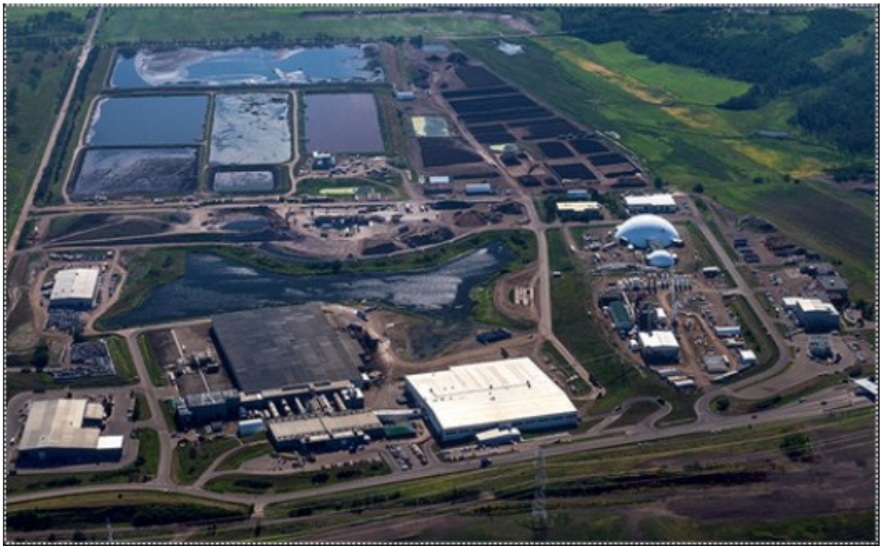
Figure 6-5 Edmonton Resource Recovery Facility
