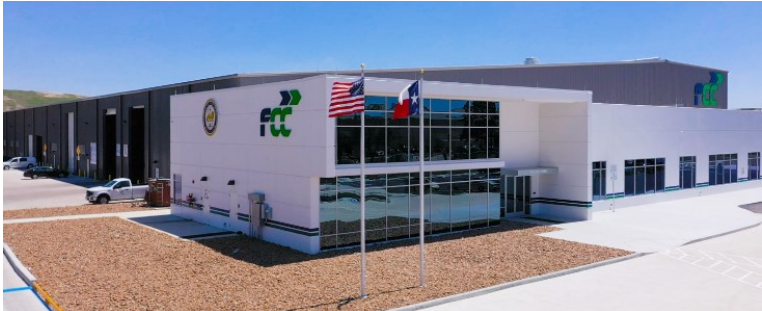
FCC Material Recovery Facility opened in 2019 to process Houston residential recyclables
