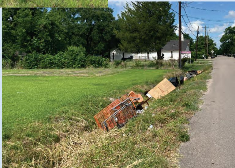
Shopping cart and other trash dumped in the bioswale, which might impair the stormwater drainage.
