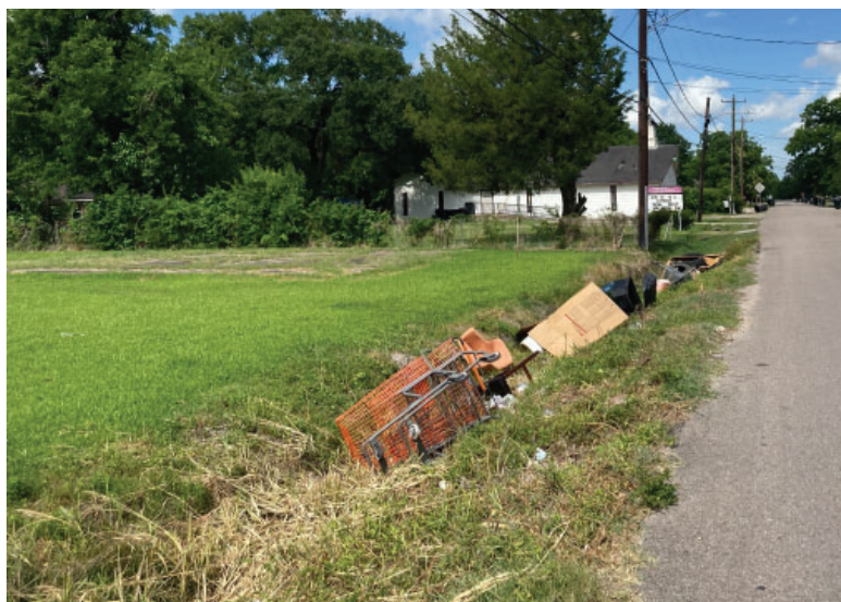
Figure 40: Shopping cart and other trash dumped in the bioswale, which might impair the stormwater drainage.
