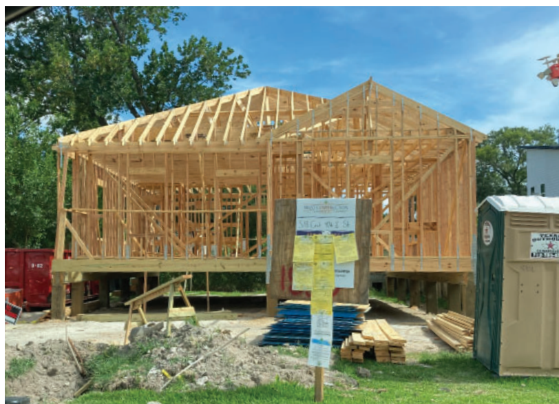
Figure 37: An new residential building under construction with elevated base.
