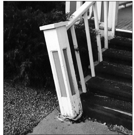
Before: A deteriorated handrail
