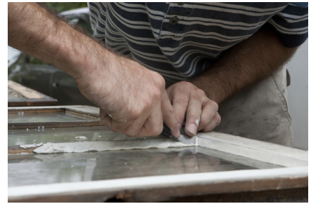
Replacing glazing putty © iStockPhoto.com/Elaine Odell
