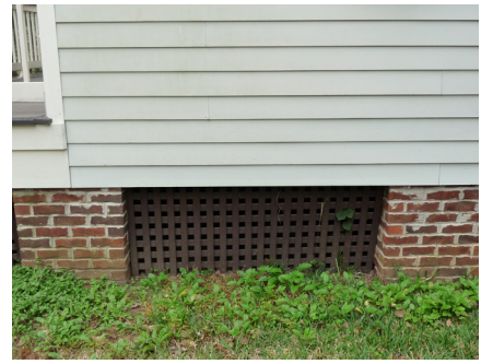
A foundation with masonry piers
