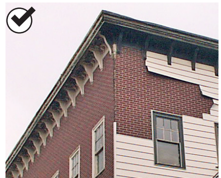
Inappropriate siding being removed from a historic brick Italianate building
