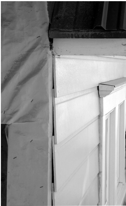
Installation of fiber-cement siding
