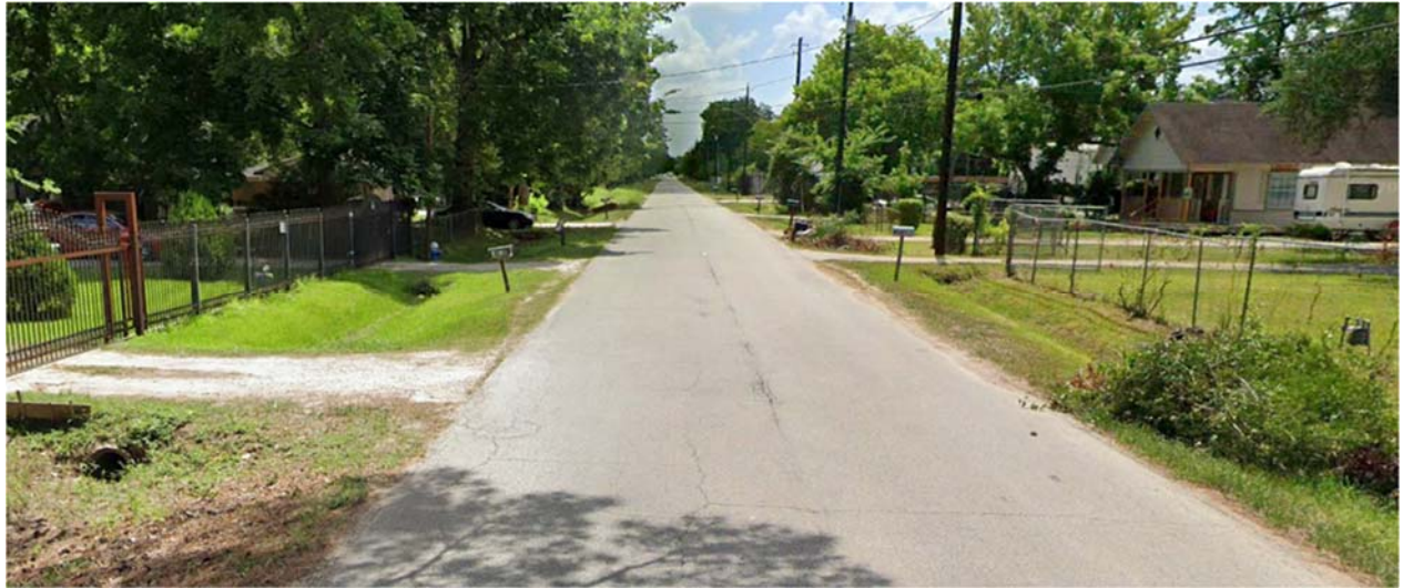
Figure 8: Existing Wilburforce Street
