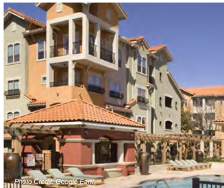
Westchase is characterized by multifamily apartment buildings.
