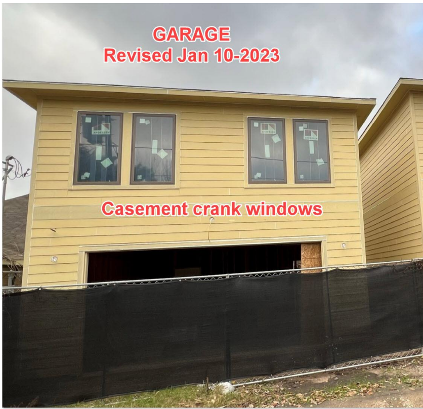
Figure 3 - Applicant Supplied Alley Elevation Photo
