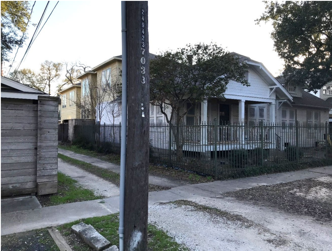
Figure 7 - View from Street down Alley January 2023
