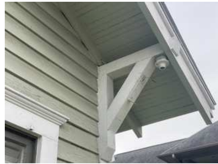
IMAGE INDICATES HISTORIC DETAILING PRESENT, EXPOSED RAFTER TAILS AND CRAFTSMAN GABLE BRACKETS
