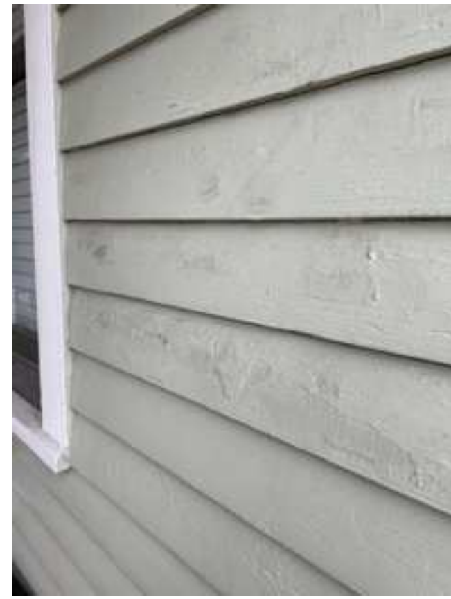
IMAGE INDICATES HISTORIC WOOD BEVEL SIDING WITH 4" REVEAL
