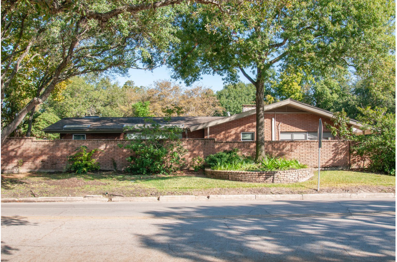
South (side) elevation facing north from Sunset Blvd.
