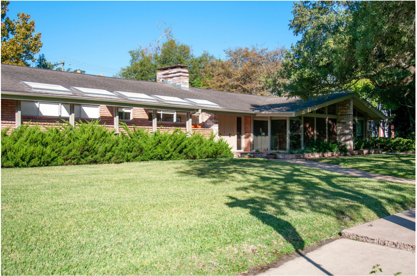
East (front) elevation facing northwest from sidewalk
