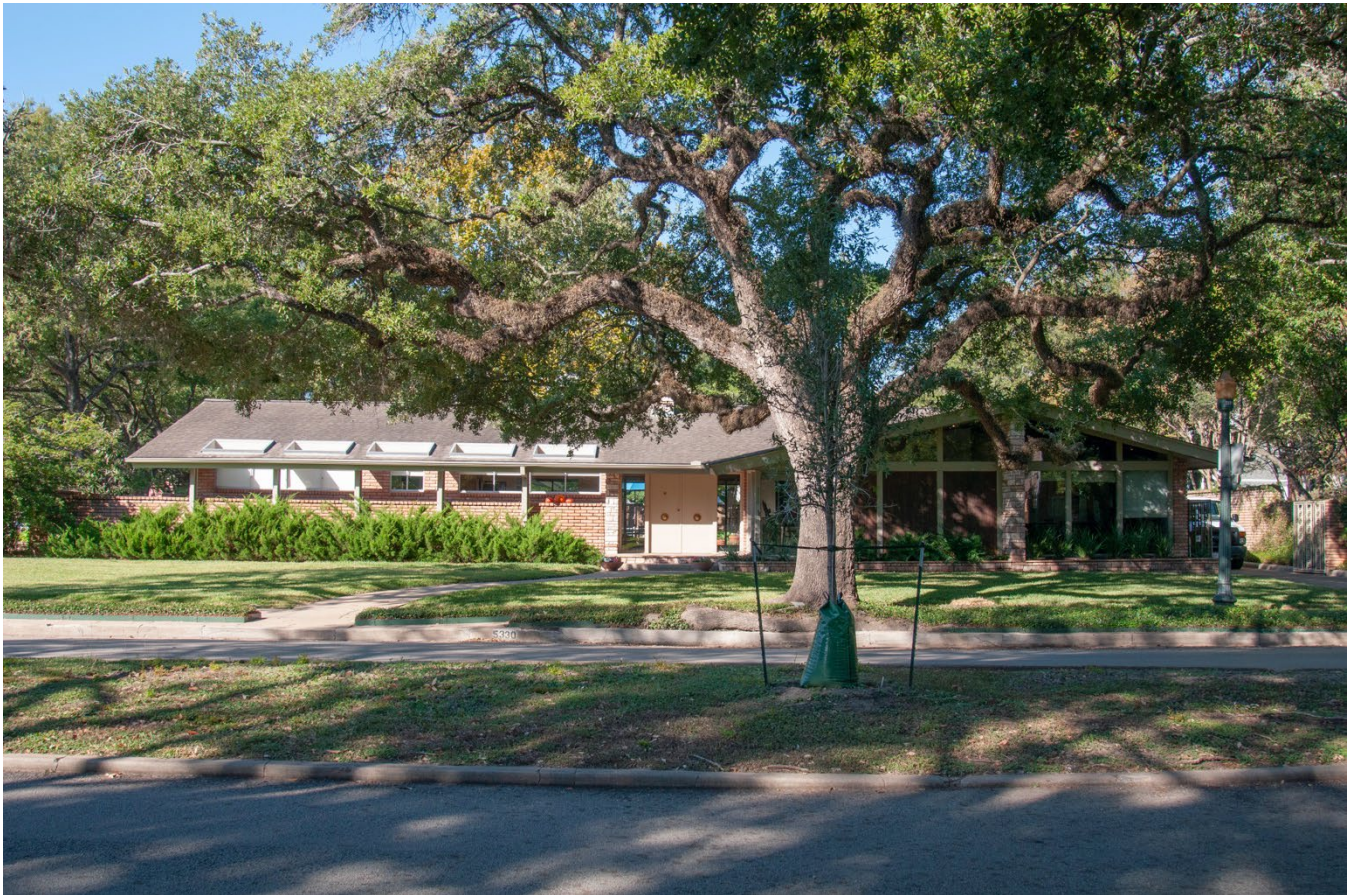
East (front) elevation facing west from Mandell St.
