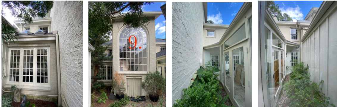
West Elevation inside of the privacy/garden wall present along the
