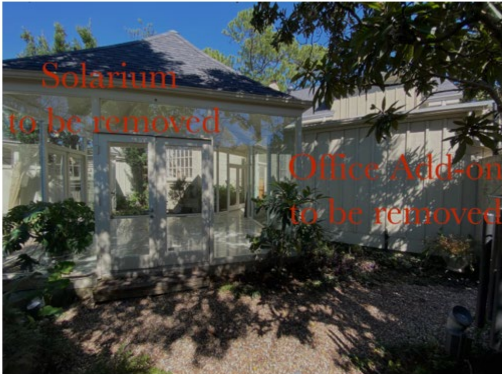
Images of Non-original Solarium and Office Add-on (circa mid-70's) Proposal to be Removed from the West Elevation of 4 W 11 th Pl
