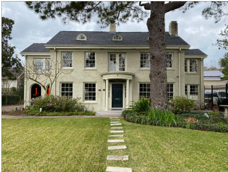
East Façade facing W 11 th Pl. *Refer to window schedule for J.
