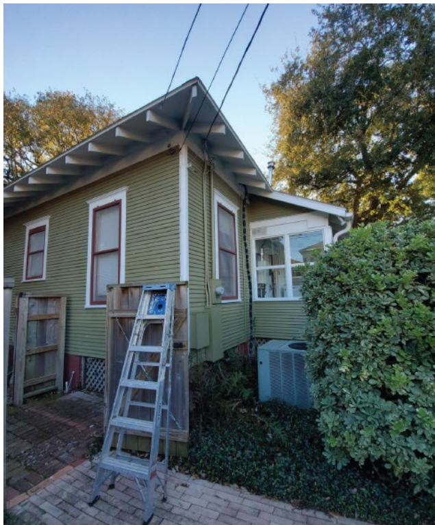
Figure 8- East Side Rear Corner
