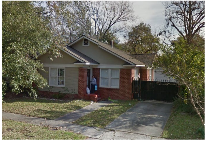
4022 Norhill Blvd – Contributing – 1929 (neighbor)
