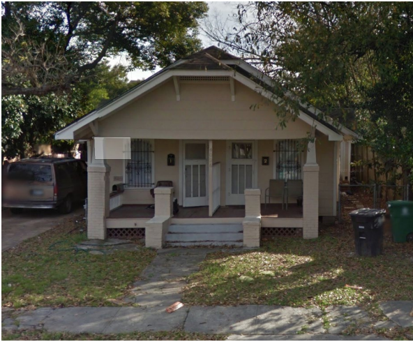
4026 Norhill Blvd – Contributing – 1929 (neighbor)
