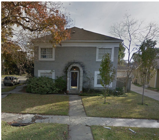
4036 Norhill Blvd – Contributing - 1930 (neighbor)
