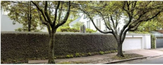
EXISTING CONDITIONS TODAY - DETACHED GUEST QUARTERS VIEWED FROM DUNLAVY ST. NOTE: EXPOSED SOUTH-FACING JULIETTE BALCONIES
