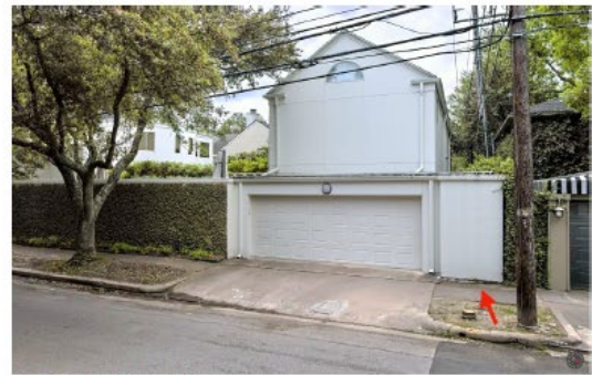
EXISTING CONDITIONS - GARAGE WALL
