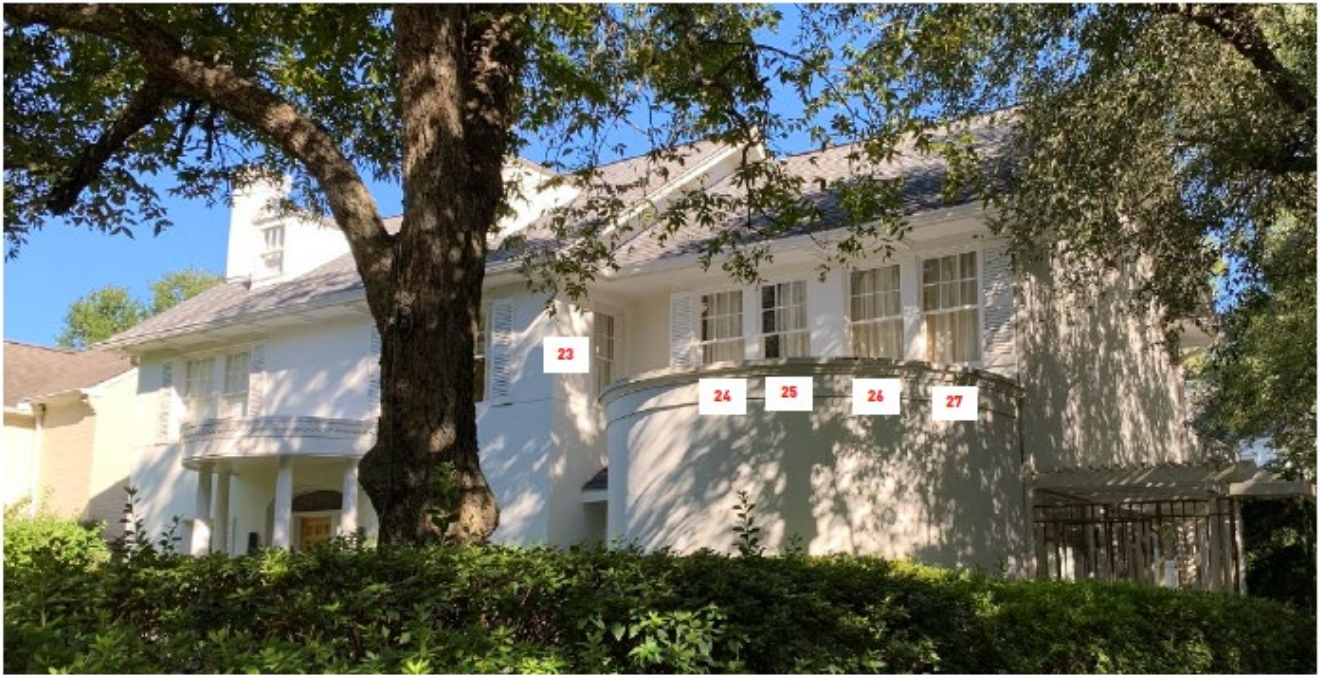
Photo of Existing Conditions with Level 2 windows to remain
