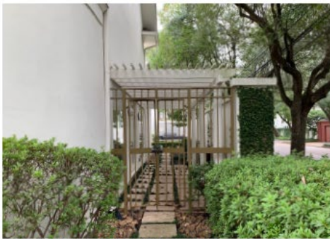
EXISTING CONDITIONS - PERIMETER WALL & METAL GATE
