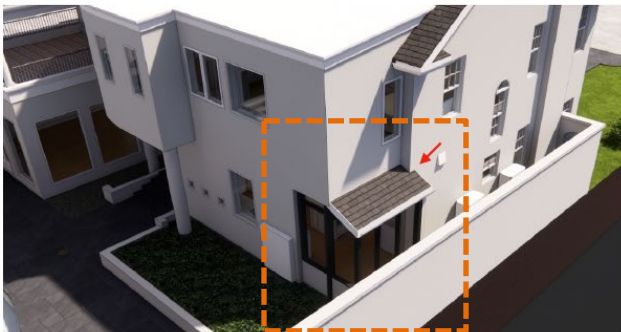
PROPOSED ROOF CONSTRUCTION OVER THE BREAKFAST ROOM. FAUX SLATE MATERIAL TO MATCH MAIN HOUSE ROOF.
