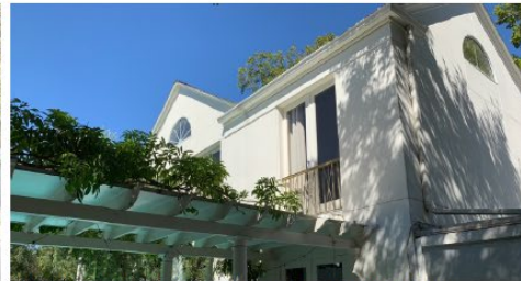
EXISTING CONDITIONS TODAY - GUEST QUARTERS VIEWED FROM BACKYARD
