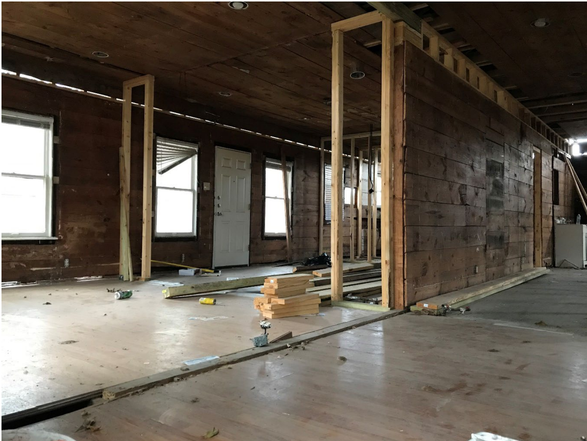
Figure 13 - Interior Shiplap Walls Intact
