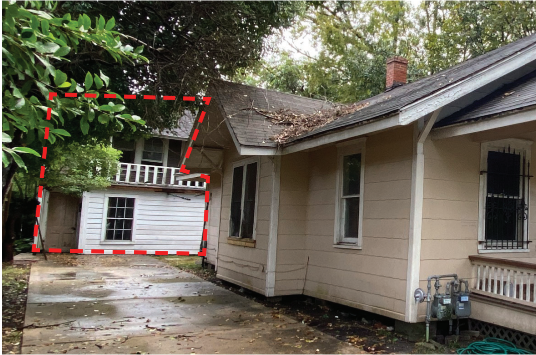
GARAGE STRUCTURE AS SEEN FROM STREET
