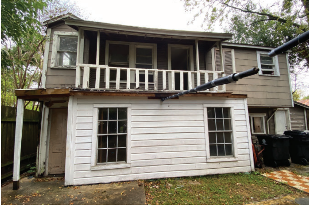
WEST ELEVATION - GARAGE STRUCTURE
