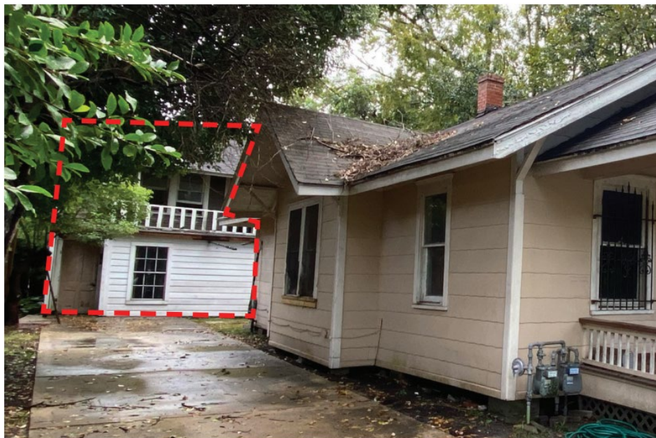
GARAGE STRUCTURE AS SEEN FROM STREET
