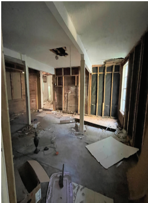
Existing First Floor at Duplex Garage Structure sits on plywood floors
