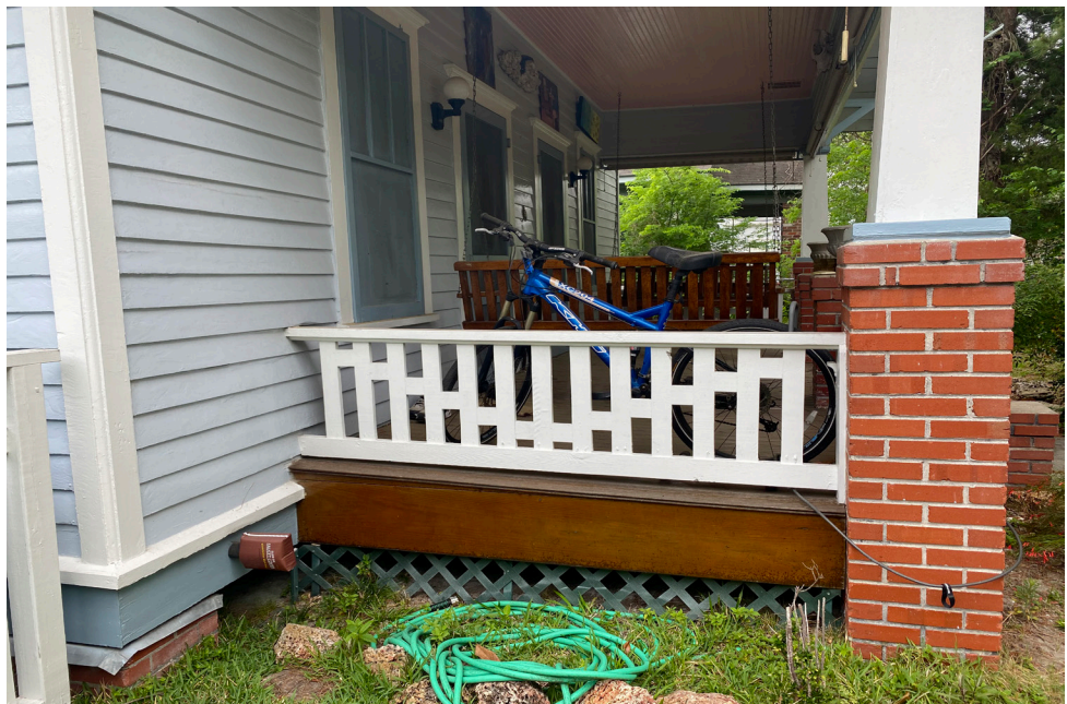
Railing Details - Front Porch
