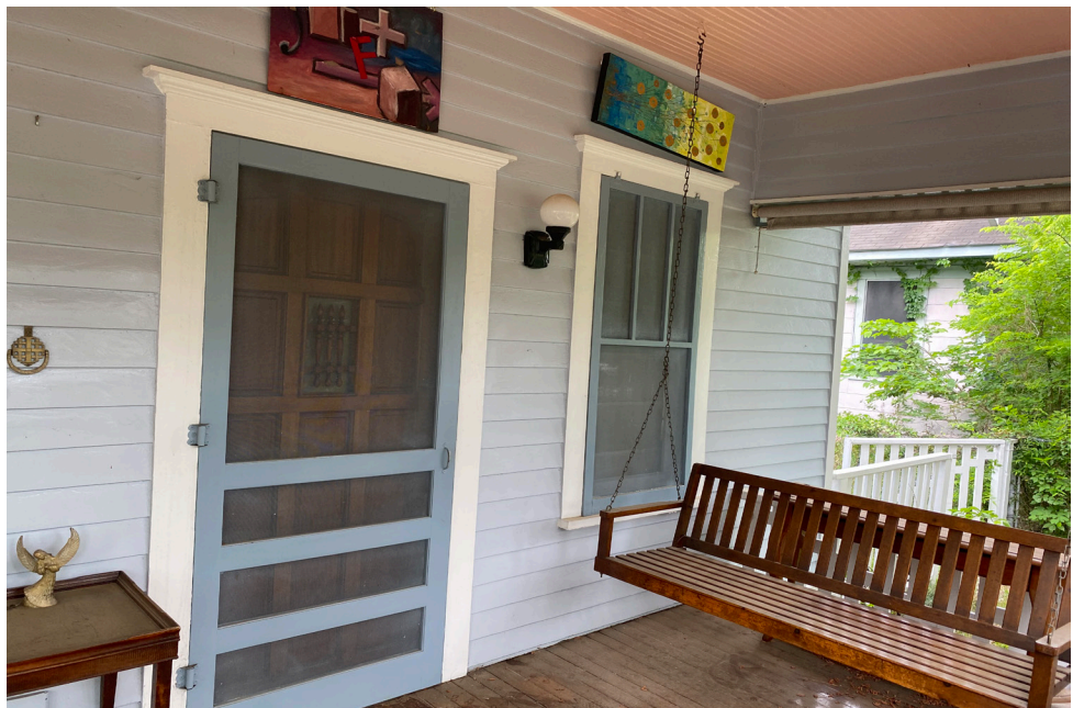
Duplex Unit 2 Entry
