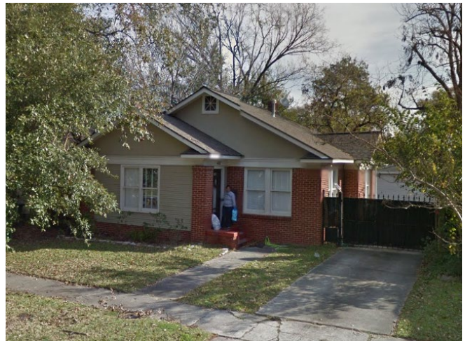
4022 Norhill Blvd – Contributing – 1929 (neighbor)
