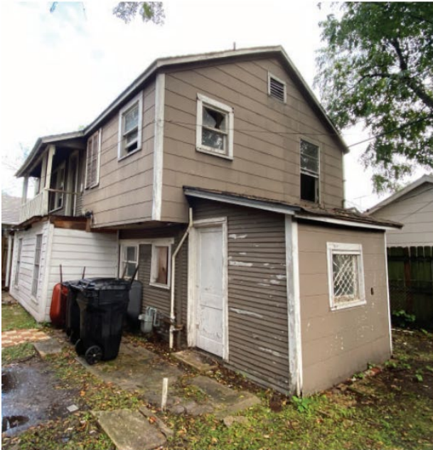
SOUTH WEST ELEVATION - GARAGE STRUCTURE
