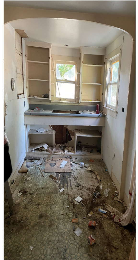
Existing First Floor Kitchen at Garage Structure
