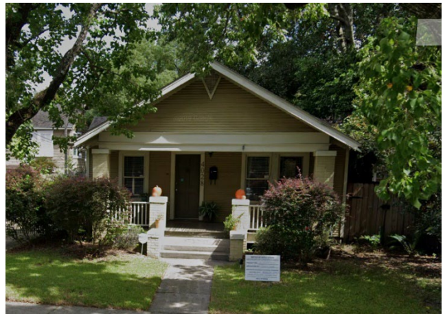
4028 Norhill Blvd – Contributing – (neighbor)
