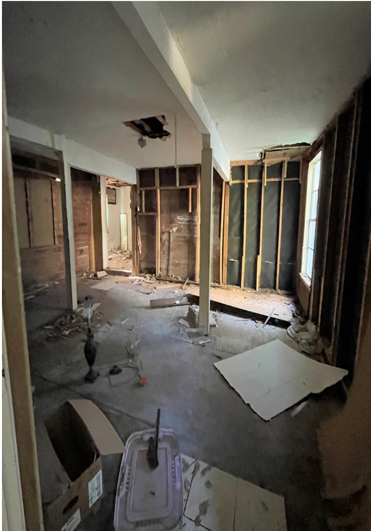
Existing First Floor at Duplex Garage Structure sits on plywood floors
