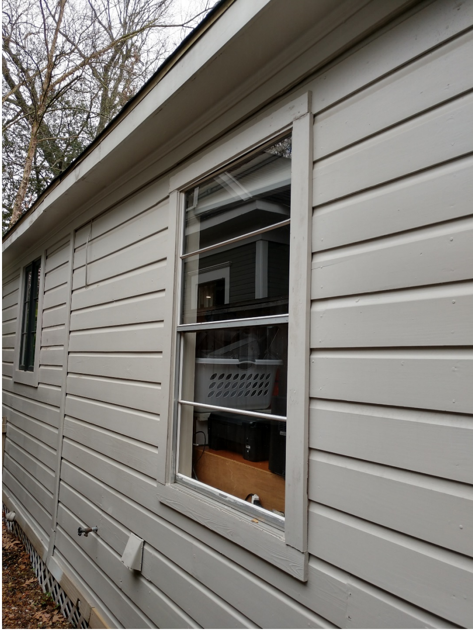
Figure 8: Northwest window to be removed
