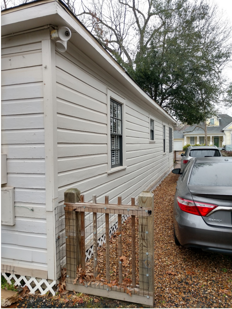
Figure 7: View of south west corner and south side
