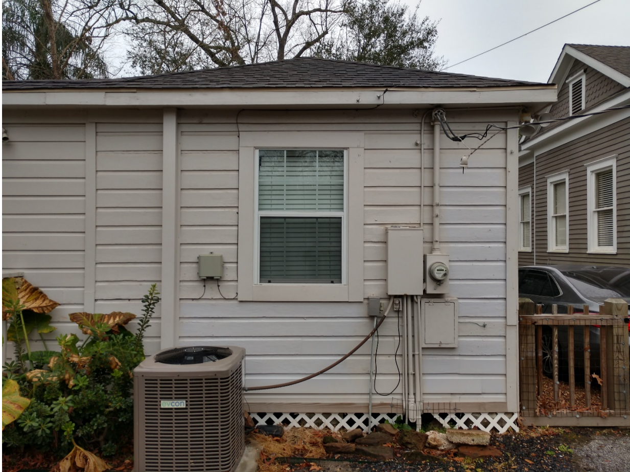
Figure 4: Back view: southwest corner
