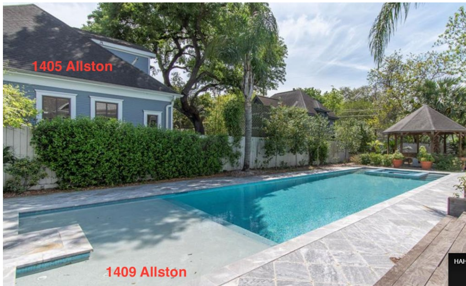
Figure 4- photo taken from HAR showing the space between both structures
