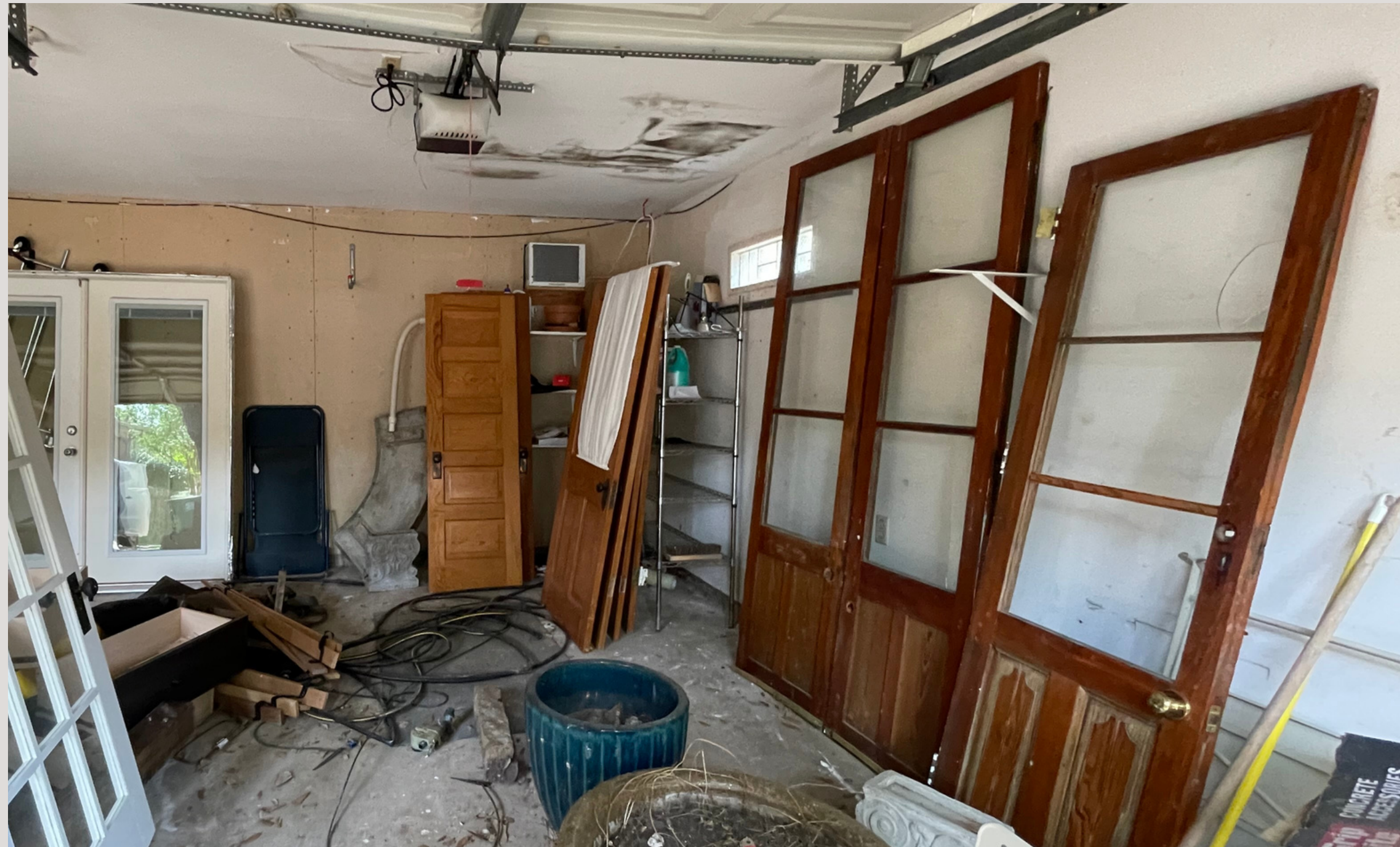
Doors left in garage that we will incorporate in the interior
