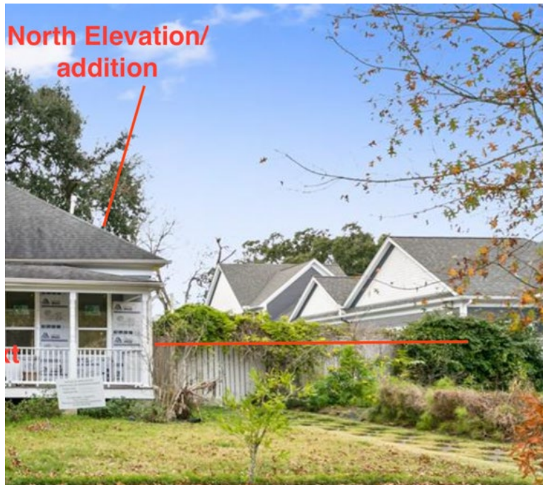
Figure 3- Google street view between both structures
