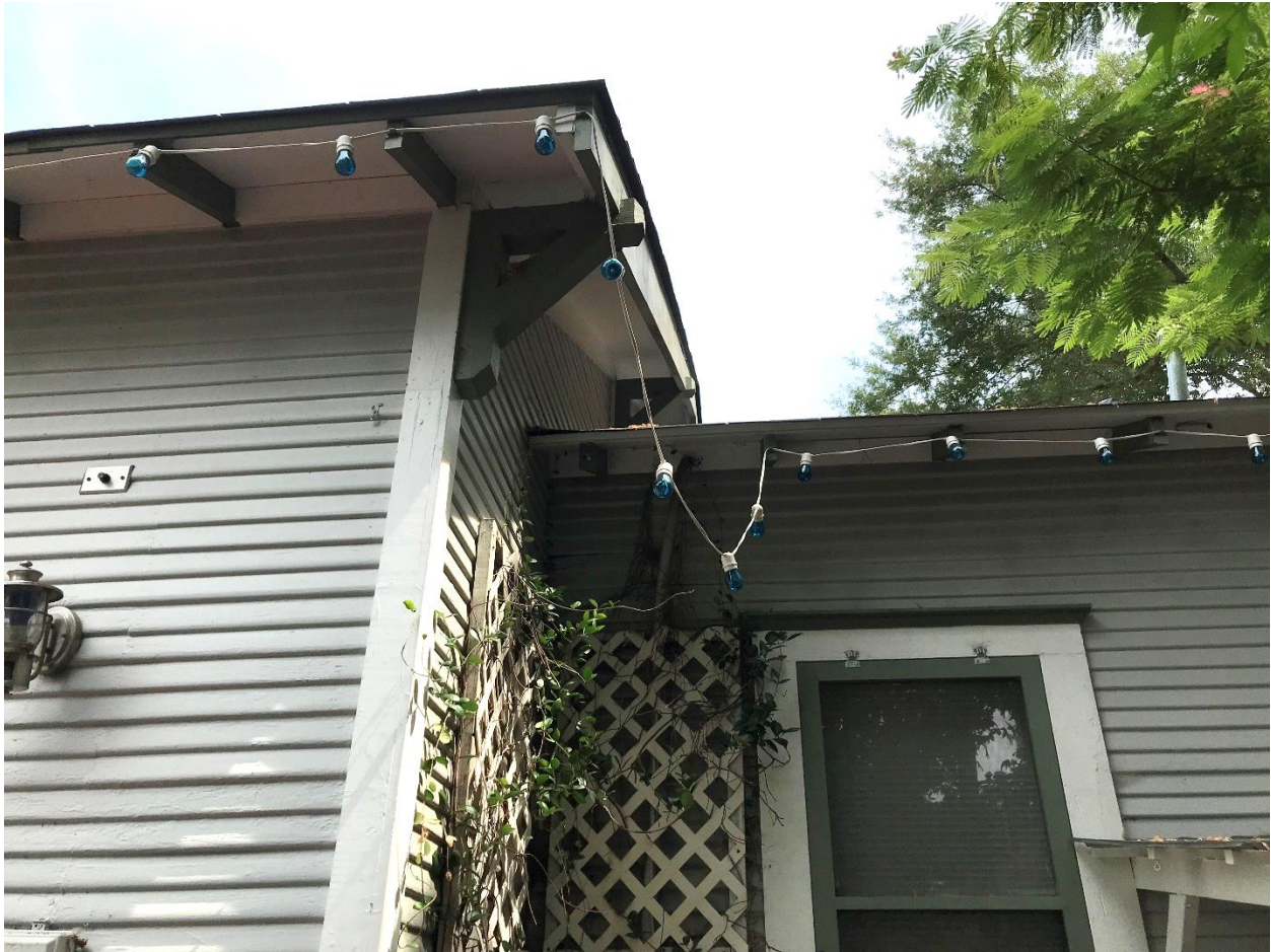
Figure 1 - Site visit - South elevation location of non-orig. addition
