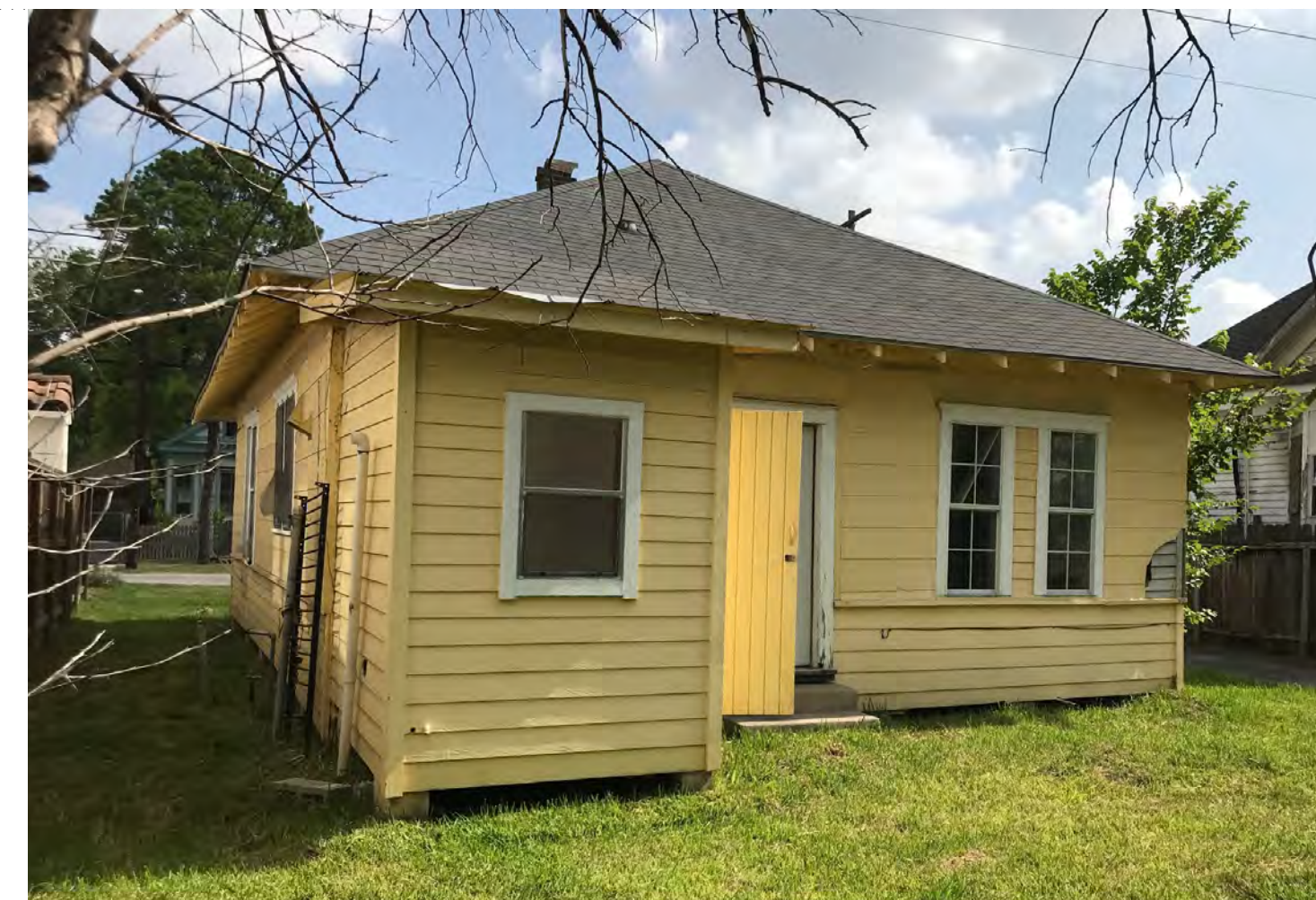
17 View from Southwest - Existing NOT TO SCALE
