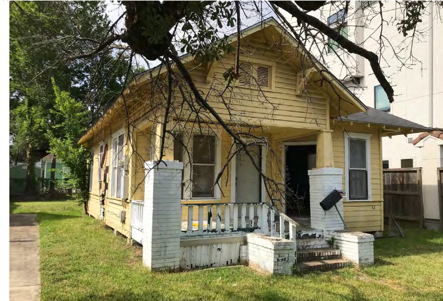
12 View from Northeast - Existing NOT TO SCALE
