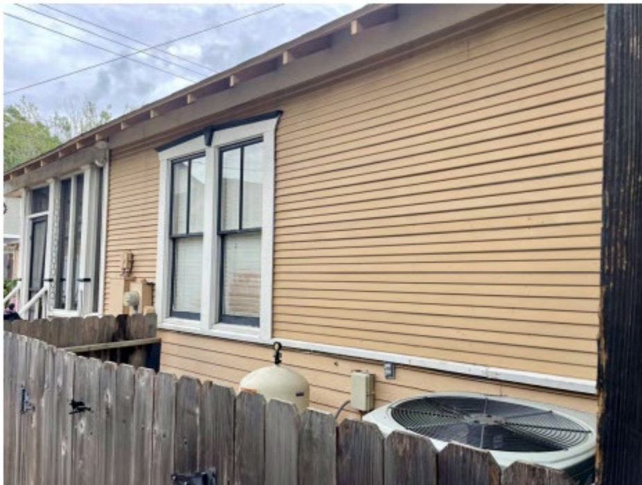
South Elevation - Behind Wood Fence
