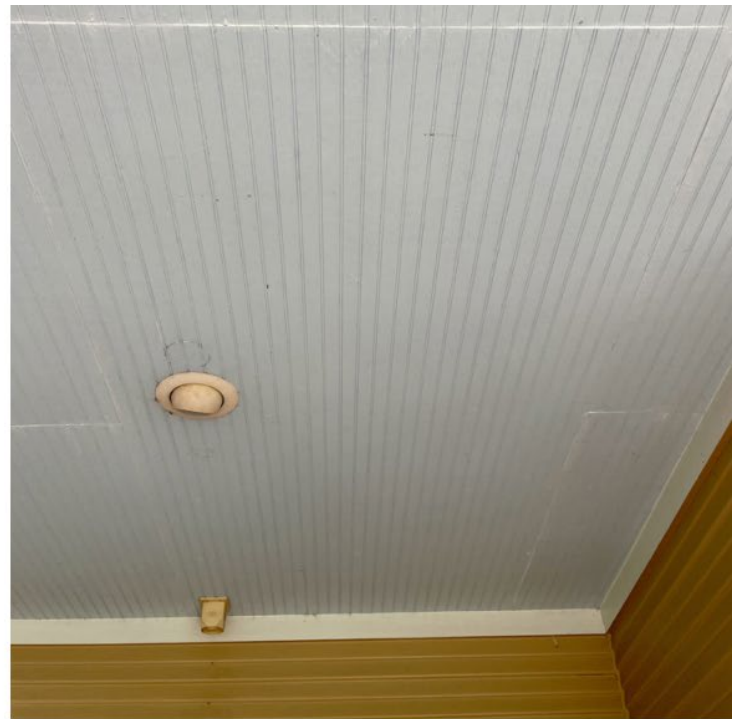
Front Porch Soffit (Non-contributing 4x8 bead board)
