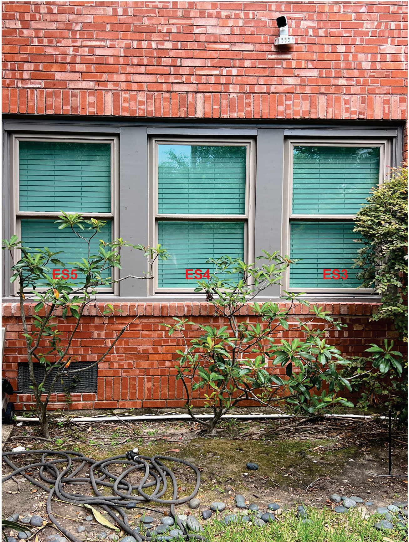
1927 South Boulevard Houston, Tx 77098 Existing Windows July 13, 2026
