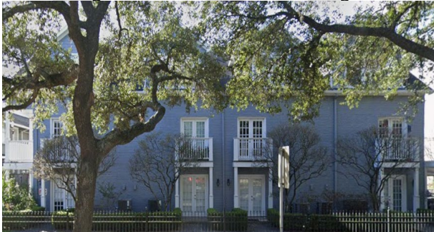
1621 Heights Blvd – Non-contributing – 2 STY
