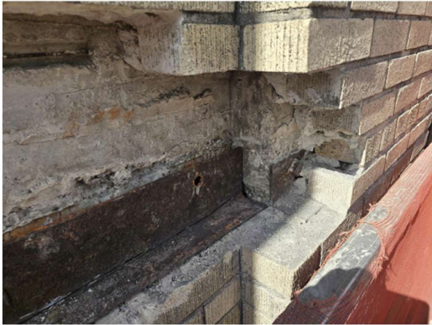
9 SHELF ANGLE (EXPOSED) AT PIER SCALE: NTS
