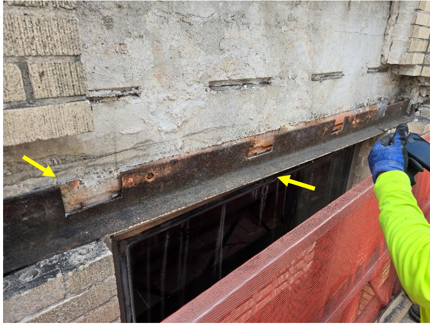
Photo No. 3. View of primary shelf angle removal in progress at cast stone spandrel. Slots in the vertical leg were cut to access the concealed weld at the vertical leg of the secondary angle behind. The concrete beam behind the shelf angle was found to be in good condition.
