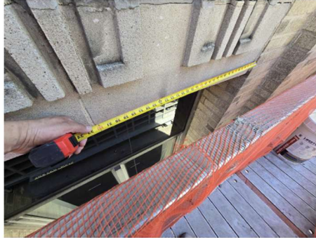
WINDOW HEADER STONE UNIT ON THE 12TH FLOOR
