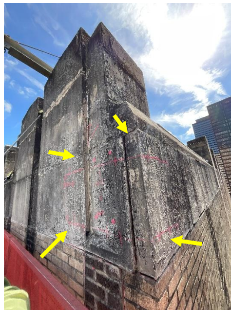
Photo No. 6. View of parapet limestone units designated for stabilization. Isolated rebuild at this section is recommended during a repair program.
