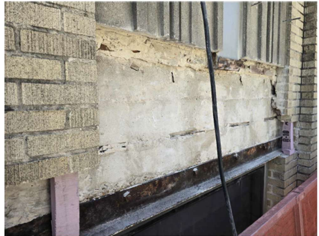
8 SHELF ANGLE (EXPOSED) AT SPANDREL SCALE: NTS
