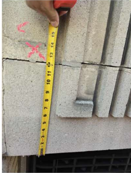
WINDOW HEADER STONE UNIT ON THE 12TH FLOOR
