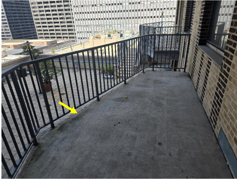
Photo No. 9. View of bare concrete balcony topside.
