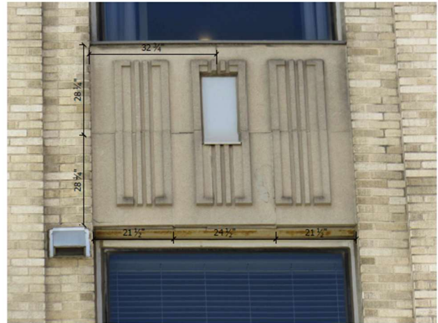
6 TYPICAL FLOOR SPANDREL SCALE: NTS
