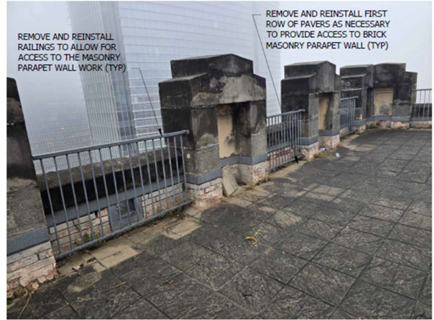
10 PARAPET BACKSIDE/ELEVATION SCALE: NTS
