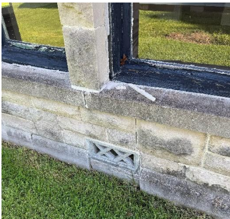
Photo 9 – Separating masonry at south elevation
