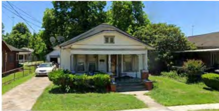
Figure 4: Picture of 202 E. 31 st ½ Street
