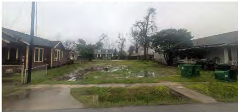
Figure 5: 202 E. 31 st ½ Street
