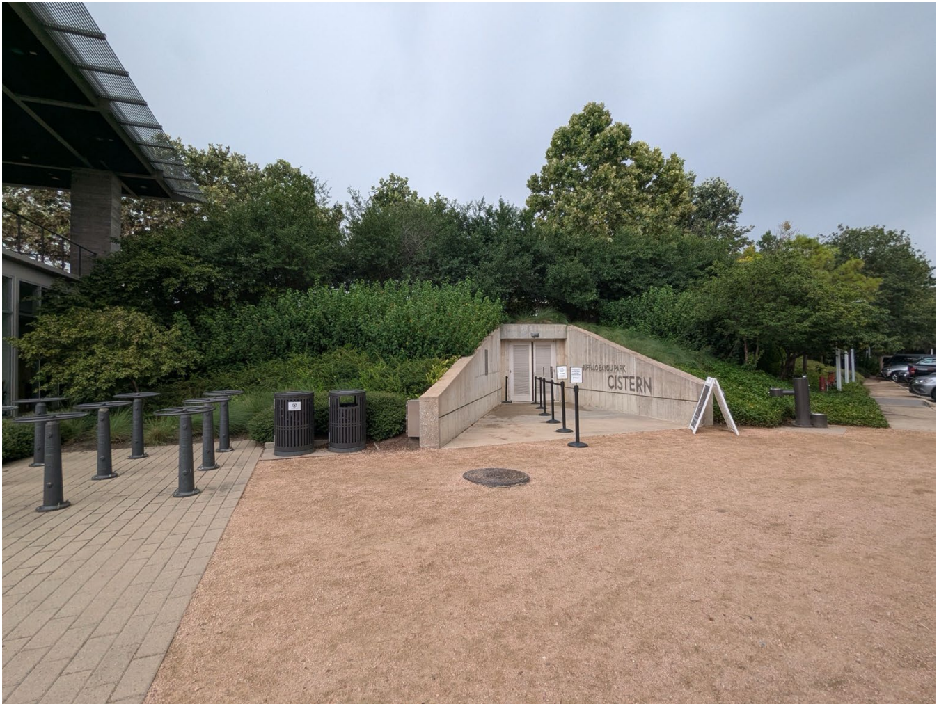
Buffalo Bayou Park Cistern entrance, facing northwest
