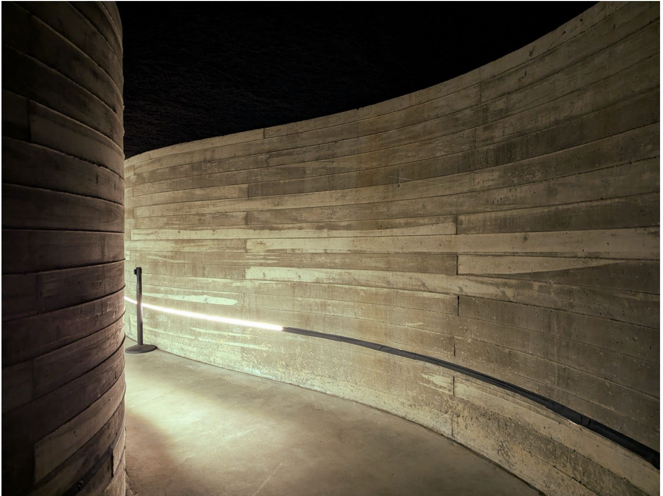
Buffalo Bayou Park Cistern entrance interior
