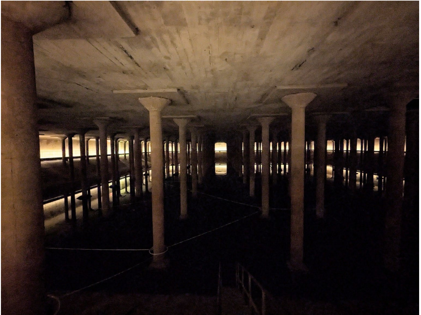
Buffalo Bayou Park Cistern interior
