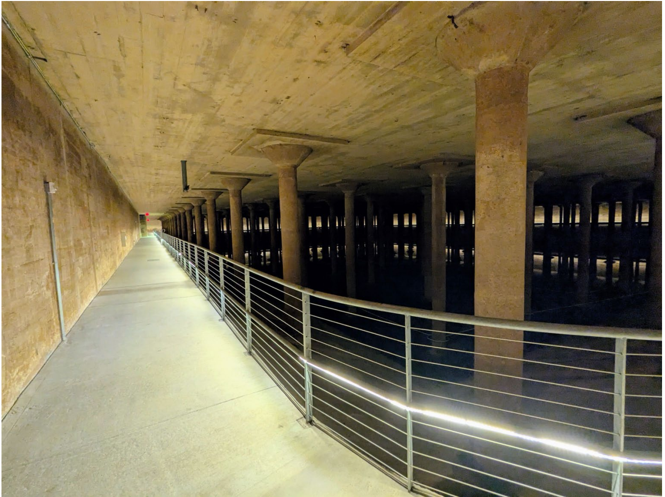
Buffalo Bayou Park Cistern interior
