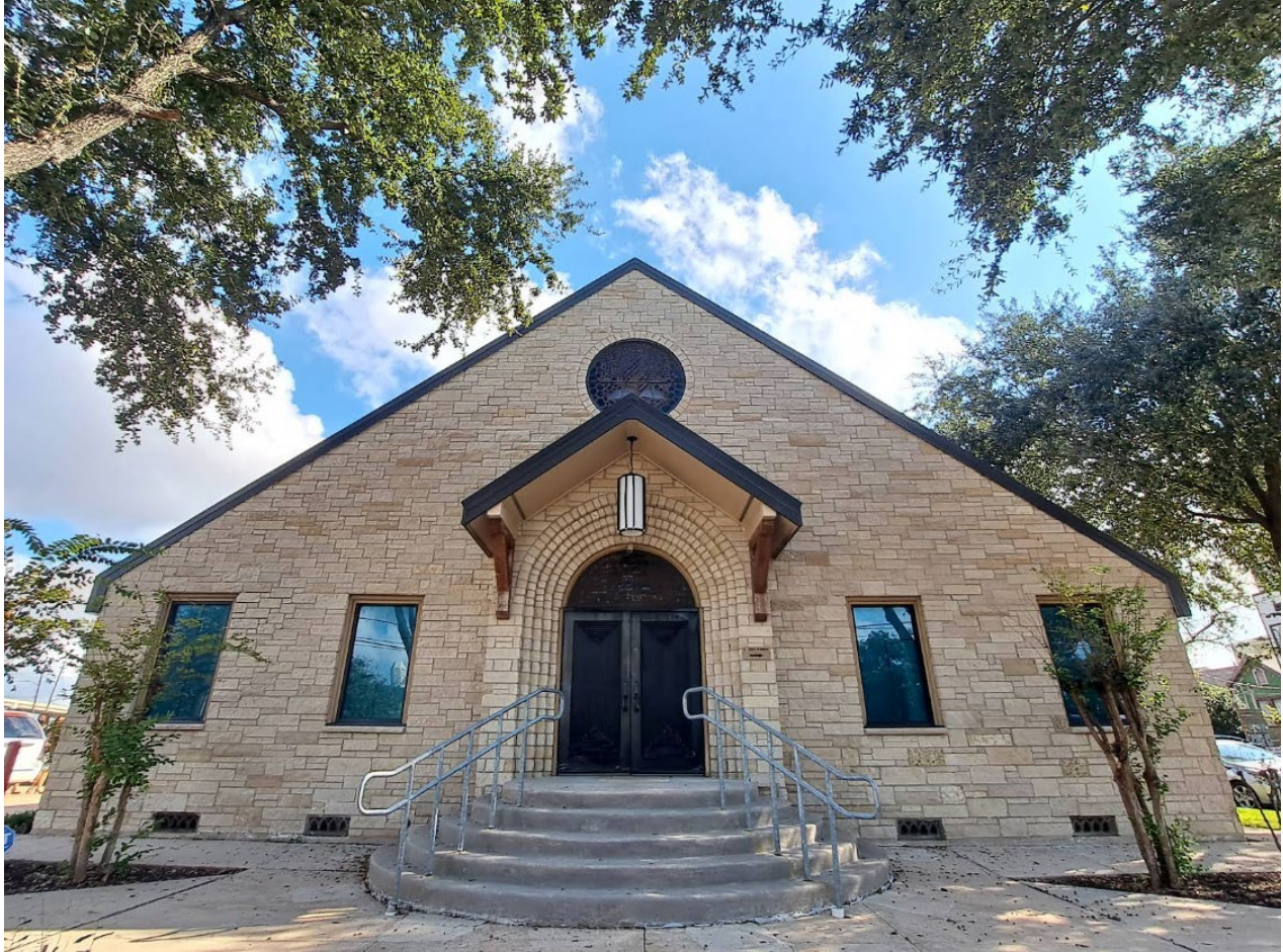
Photo 1 Southeast (Front) Façade
