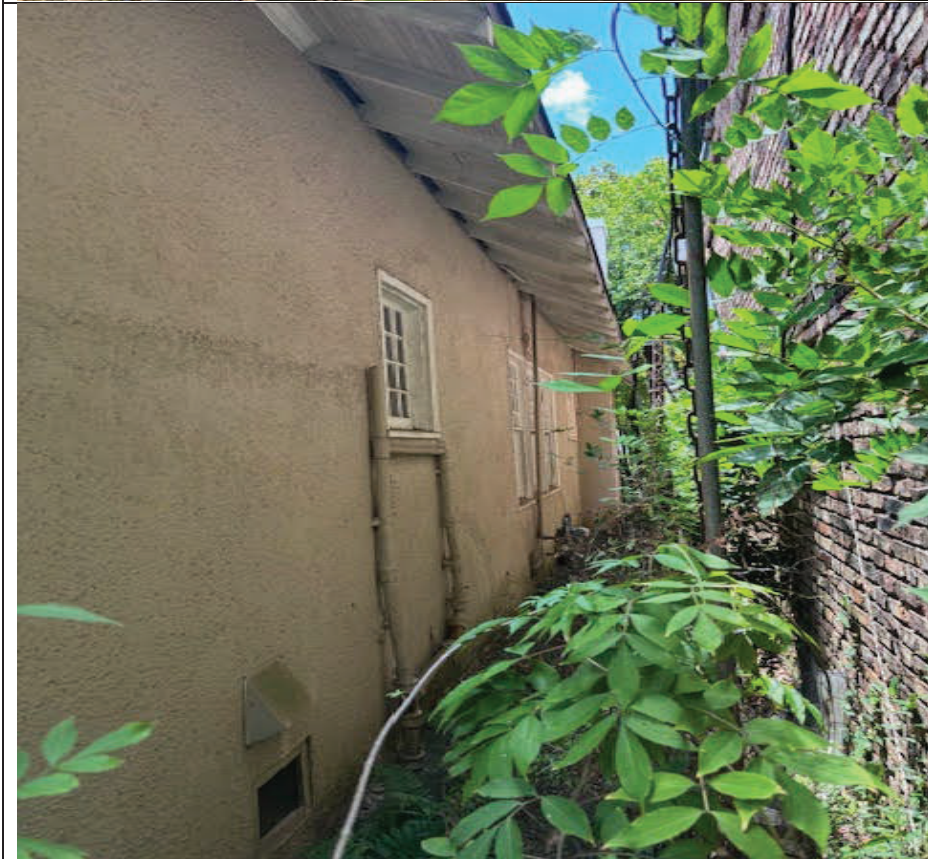
West elevation From back
