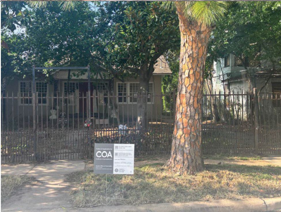
South elevation From street Showing the sign too
