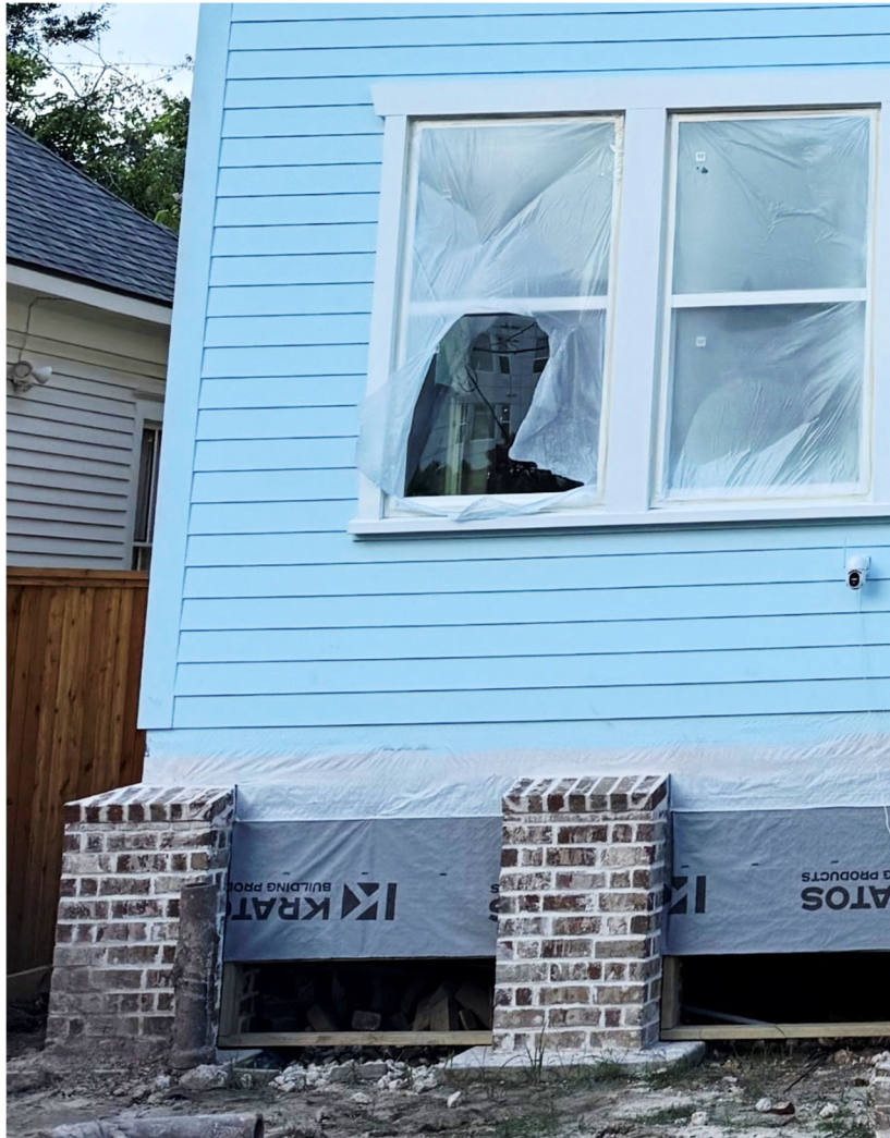
Brick piers have been exposed; flared skirting of siding has been removed.
