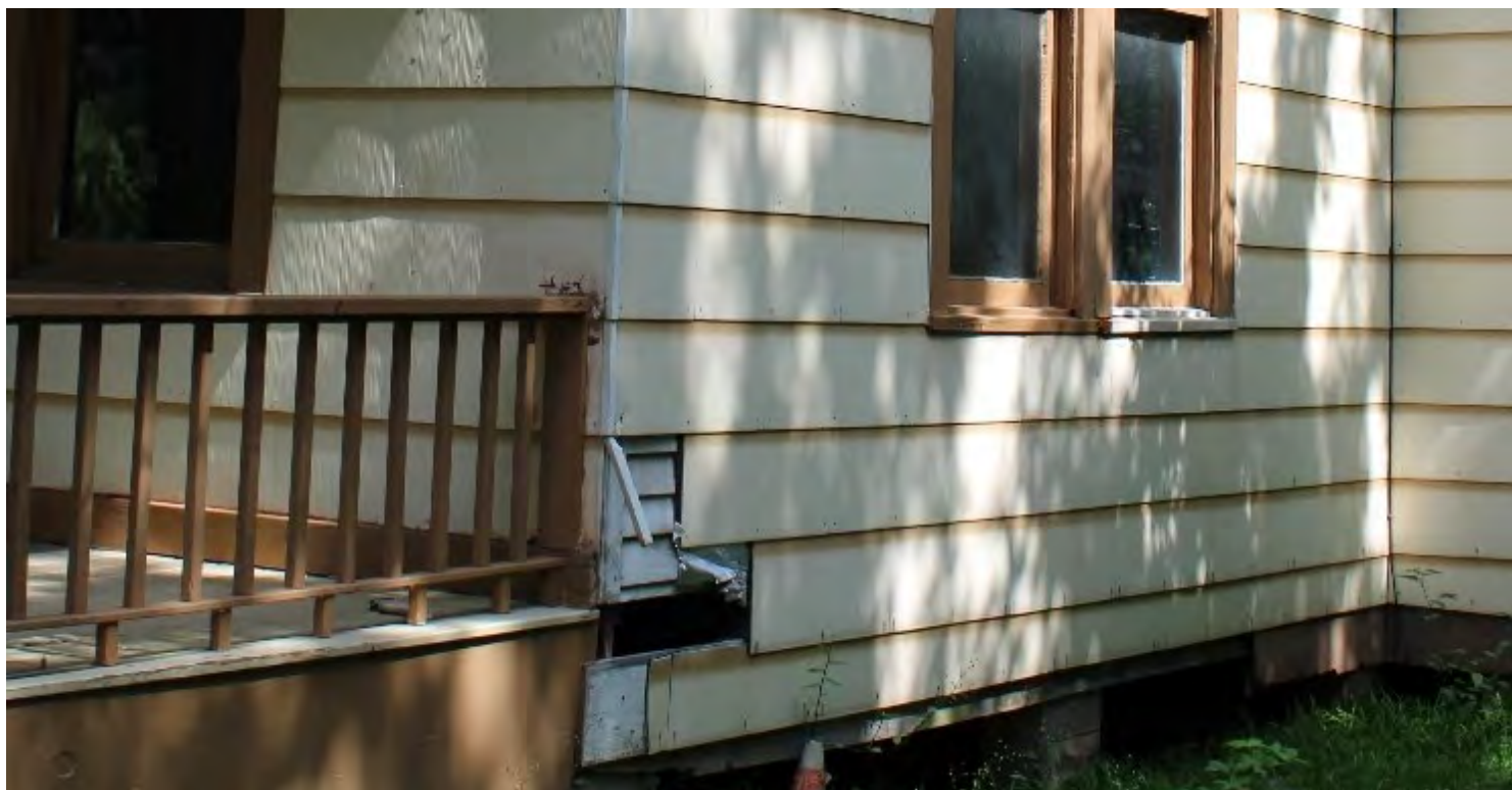
Figure 4 - Image of Beveled Siding Under Synthetic
