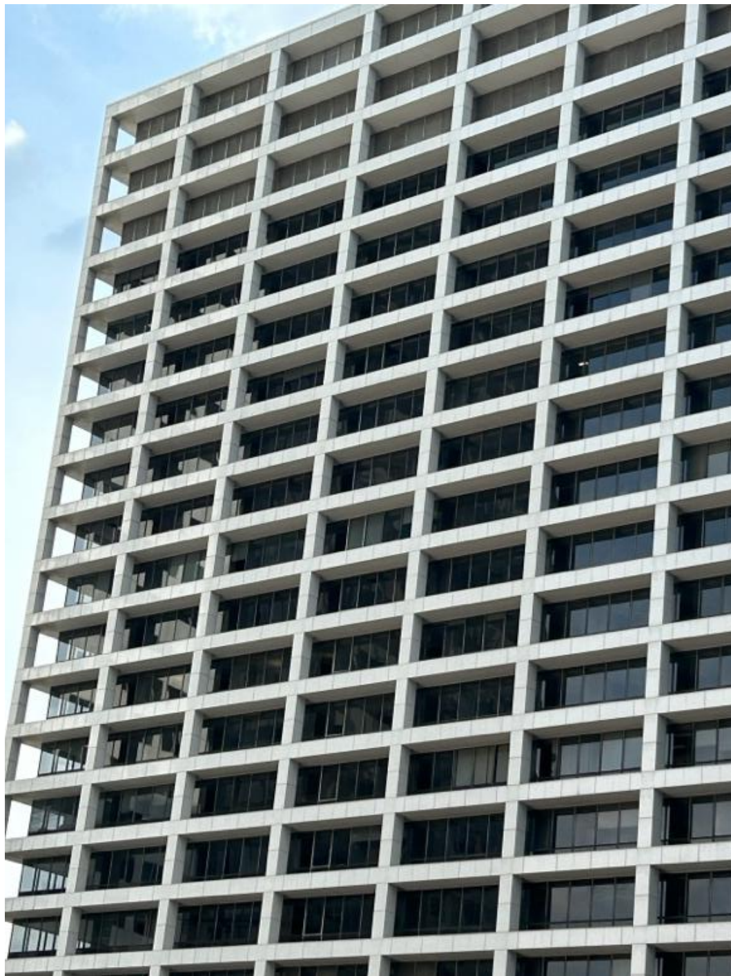
Photo 4. Northeast (McKinney Street) elevation, façade detail, operable side hinged windows for maintenance access visible in fourth bay from left, view south
