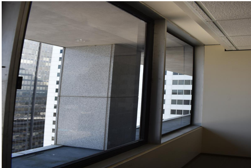
Photo 28. Floor 29, typical operable side hinged window and latch, view north
