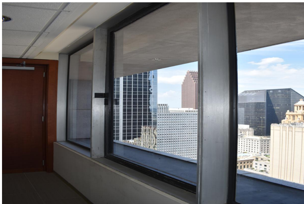
Photo 28. Floor 29, typical operable side hinged window and latch, view north
