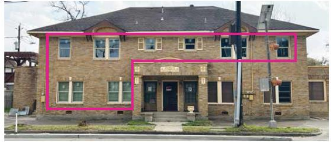
Partially Installed New Windows
