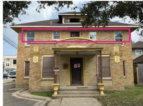
Partially Installed New Windows
