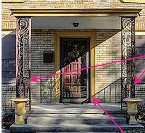
Existing Door Dimension: 36" W x 80" H Material: Wood with Glass, and Storm Door
