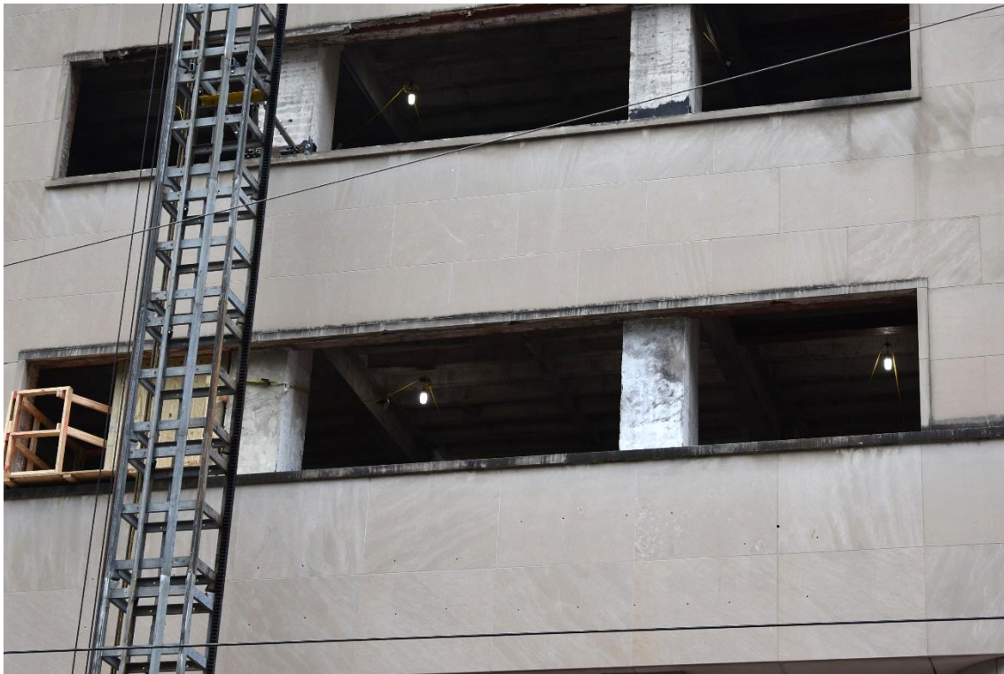
Photo 16: East elevation facing Main Street, third and fourth floor; view west.
