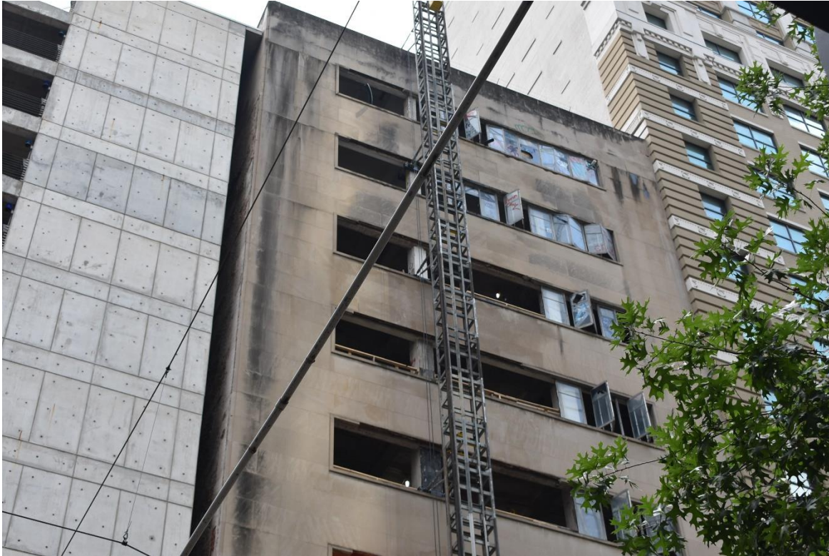
Photo 12: East elevation facing Main Street, upper floors; view northwest.
