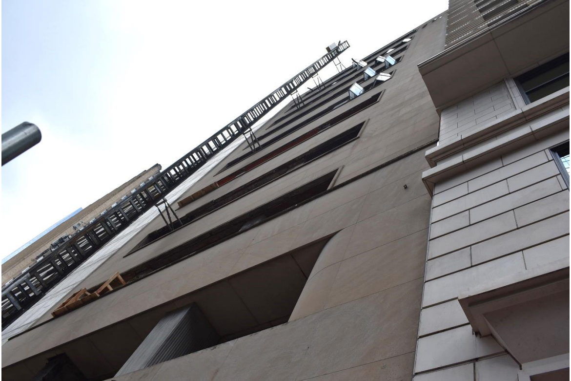
Photo 7: East elevation facing Main Street; view southwest.
