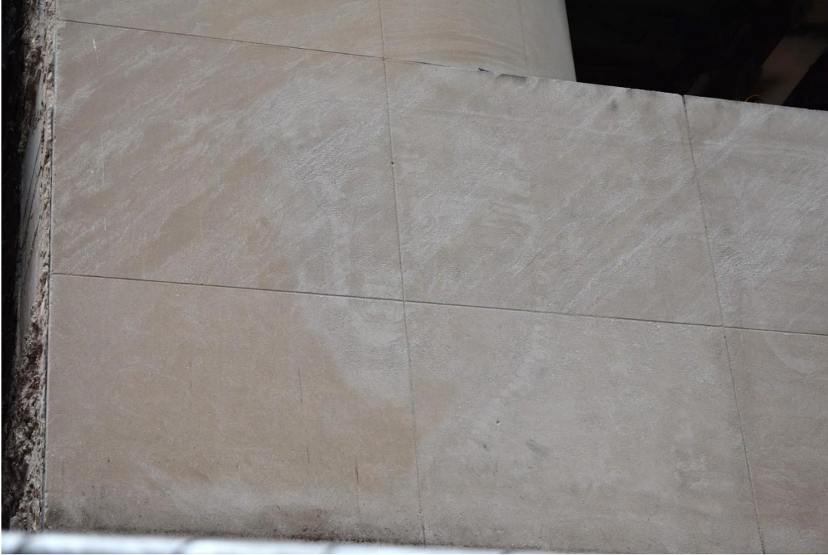
Photo 21: East elevation facing Main Street, detail of limestone façade; view north.
