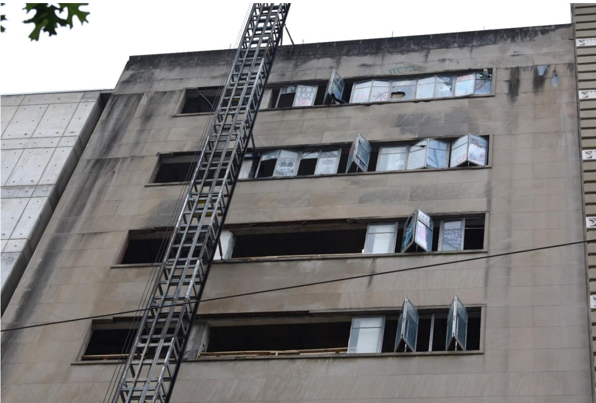
Photo 13: East elevation facing Main Street, upper floors; view west.
