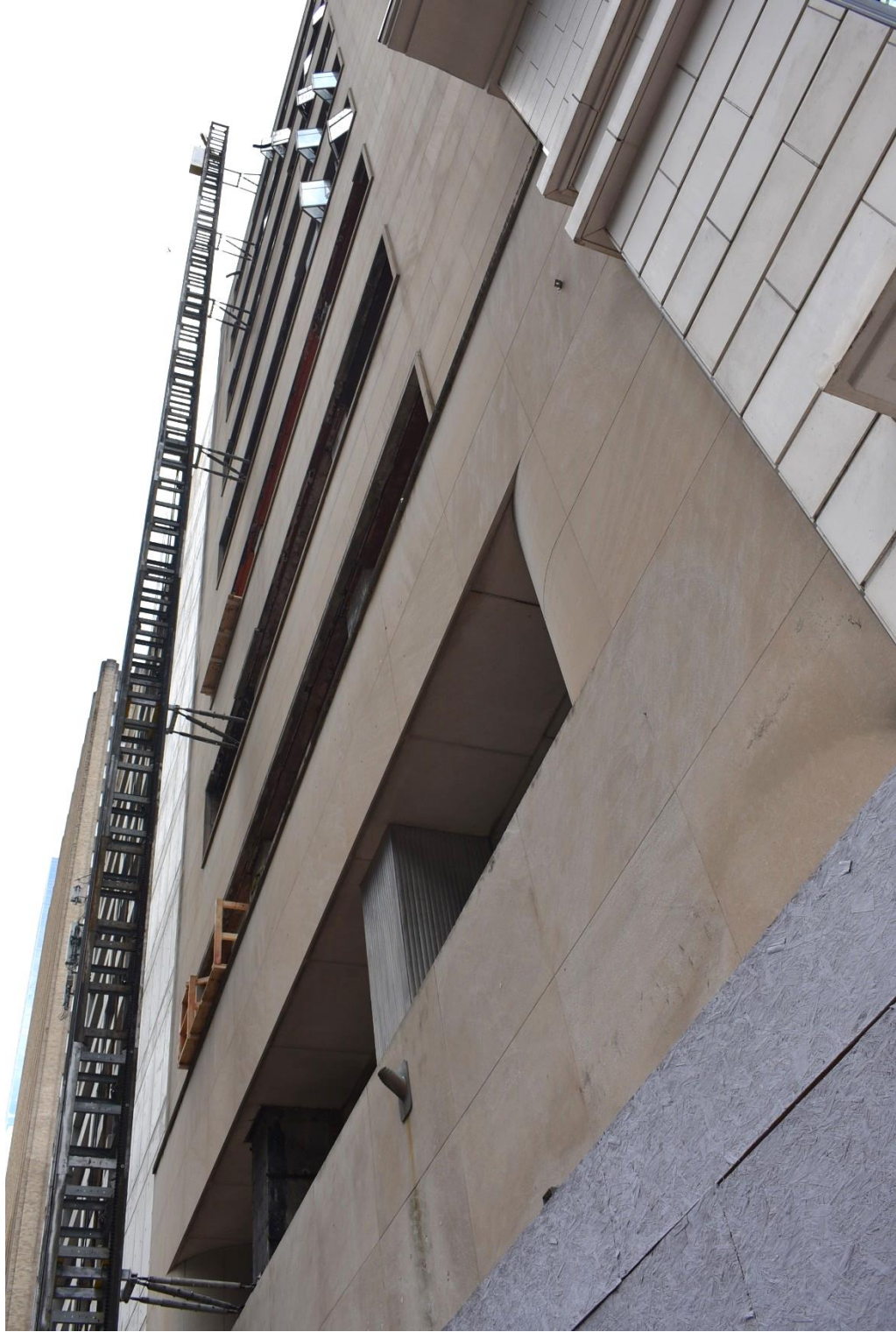
Photo 5: East elevation facing Main Street; view southwest.
