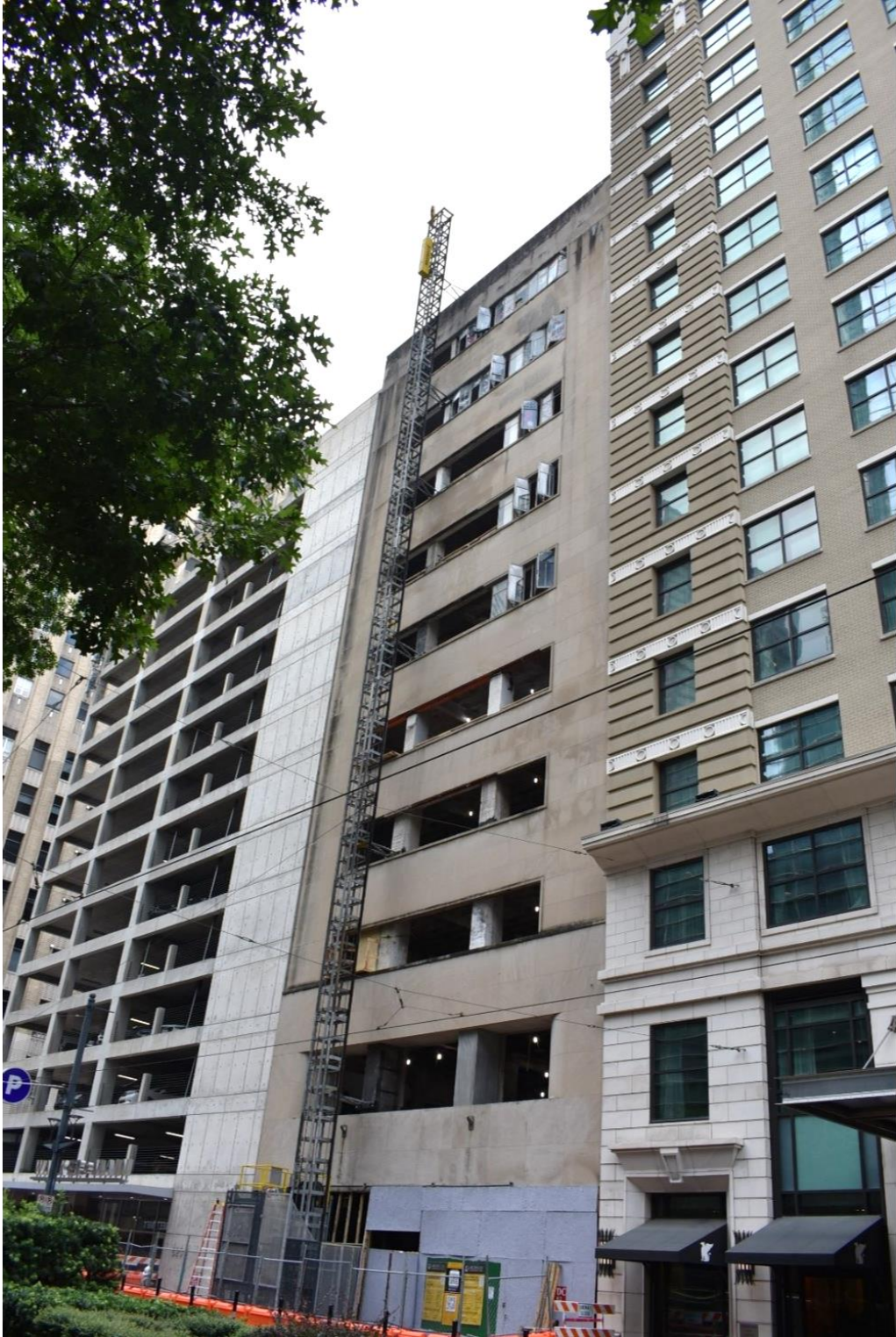
Photo 2: East elevation facing Main Street; view southwest.
