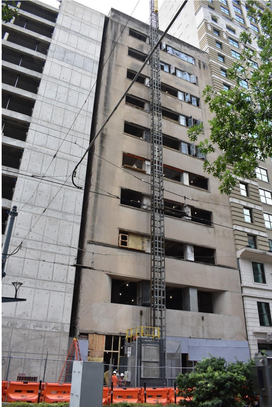
Photo 1: East elevation facing Main Street; view north.
