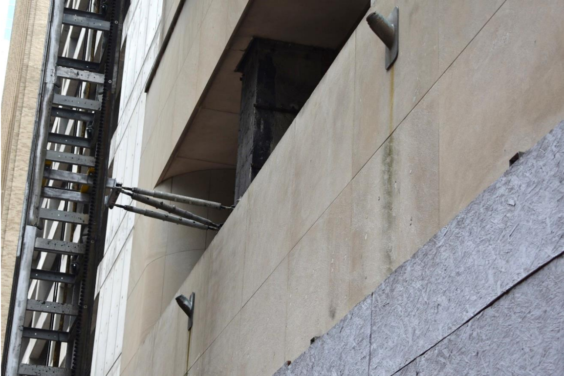
Photo 19: East elevation facing Main Street, second floor exterior; view southwest.
