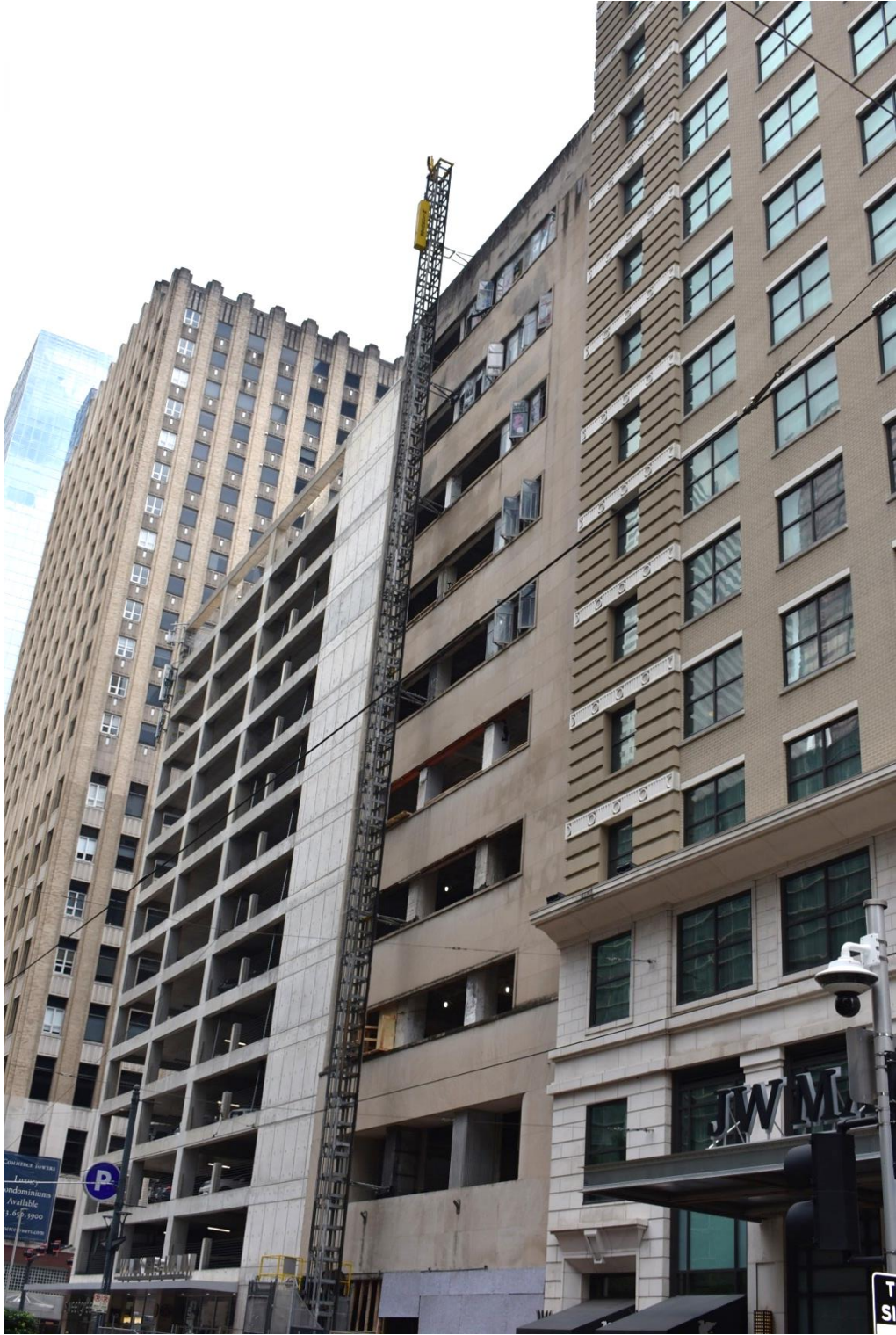
Photo 4: East elevation facing Main Street; view southwest.
