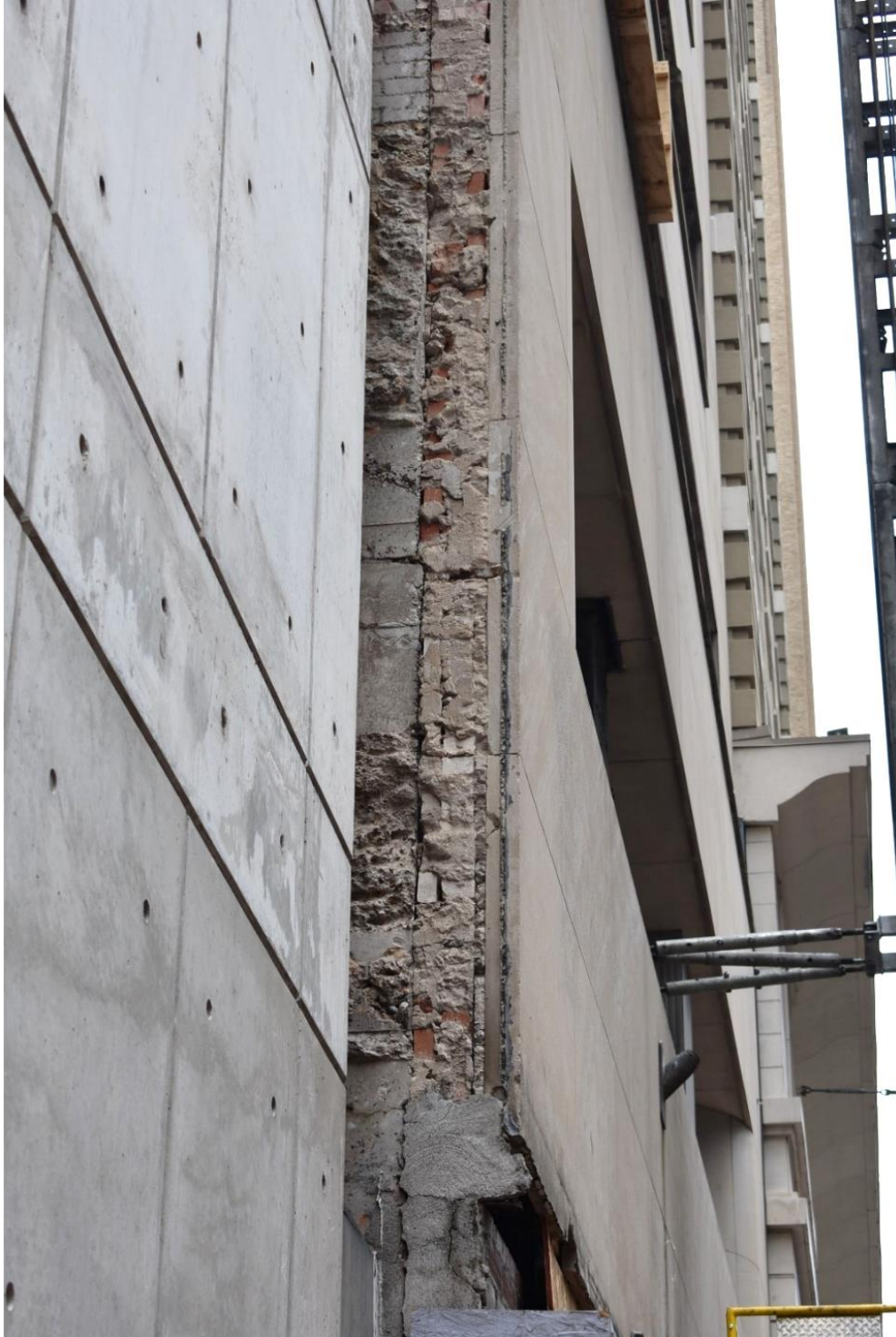
Photo 10: East elevation facing Main Street, detail view of exterior limestone and brick; three-quarter view north.
