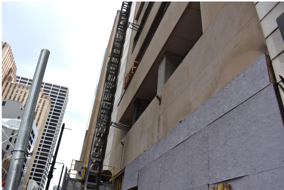
Photo 15: East elevation facing Main Street, lower floors; view southwest.
