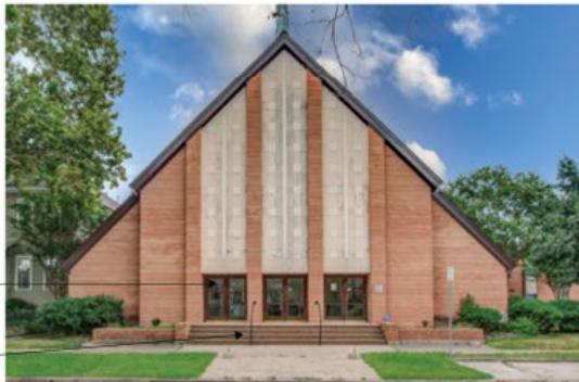
BUILDING 1 - (WEST ELEVATION) REHABILITATION
