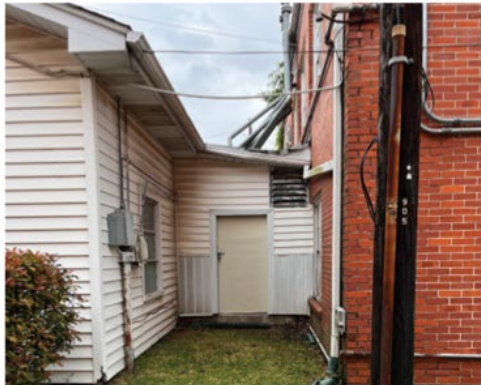
South Elevation of Building 2 Addition
