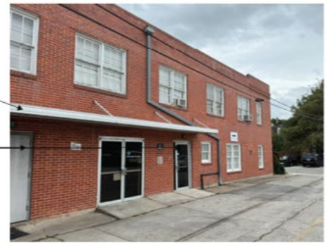
BUILDING 2 - (WEST ELEVATION) REHABILITATION
