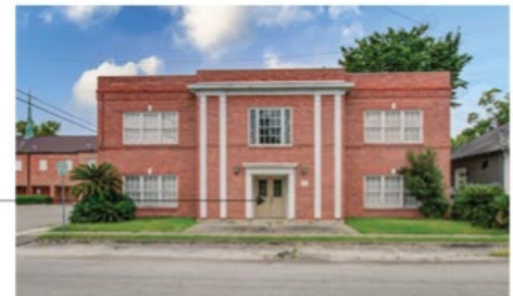
BUILDING 2 - (SOUTH ELEVATION) REHABILITATION
