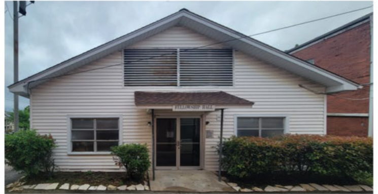
West Elevation of Building 2 Addition
