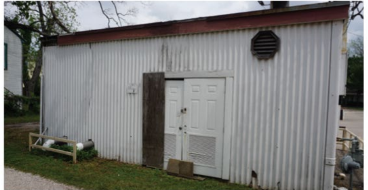
West Elevation of Building 3
