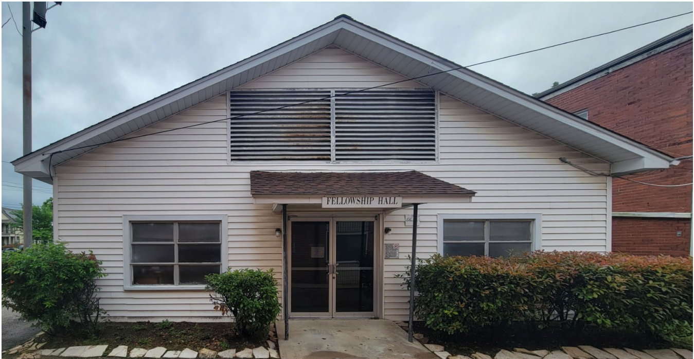
Figure 3- noncontributing structure to be demolished.
