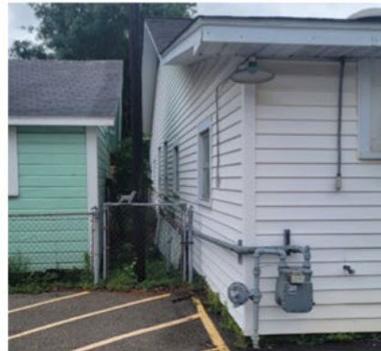
East Elevation of Building 2 Addition
