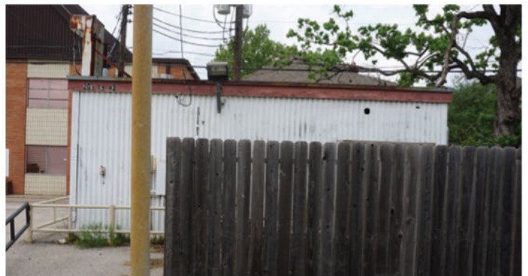
East Elevation of Building 3
