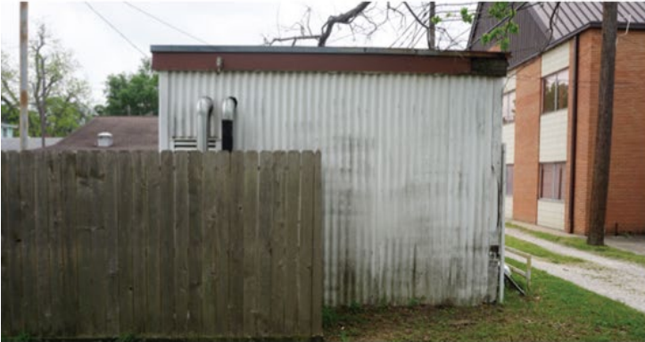
North Elevation of Building 3
