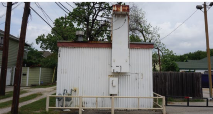
South Elevation of Building 3
