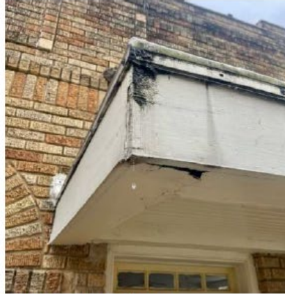
Photo 2 – Water damage
