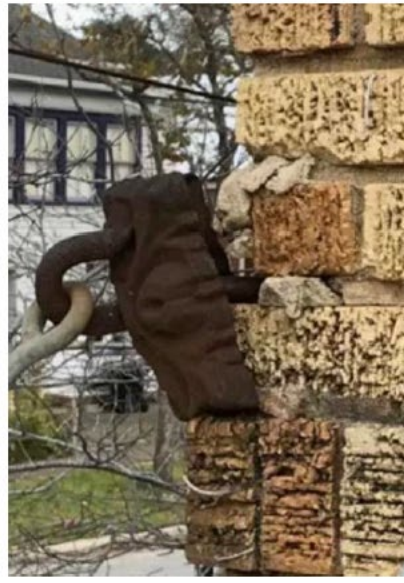
Photo 6 – Failing attachment
