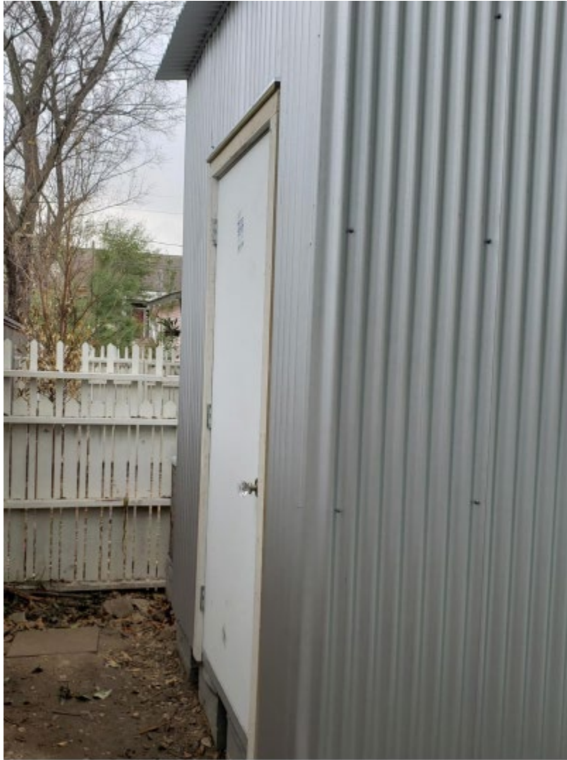
Figure 2- STORAGE BUILT WITH NO PERMIT, NO NEED FOR COA AS ITS EXEMPT AND CAN'T BE SEEN FROM ROW
