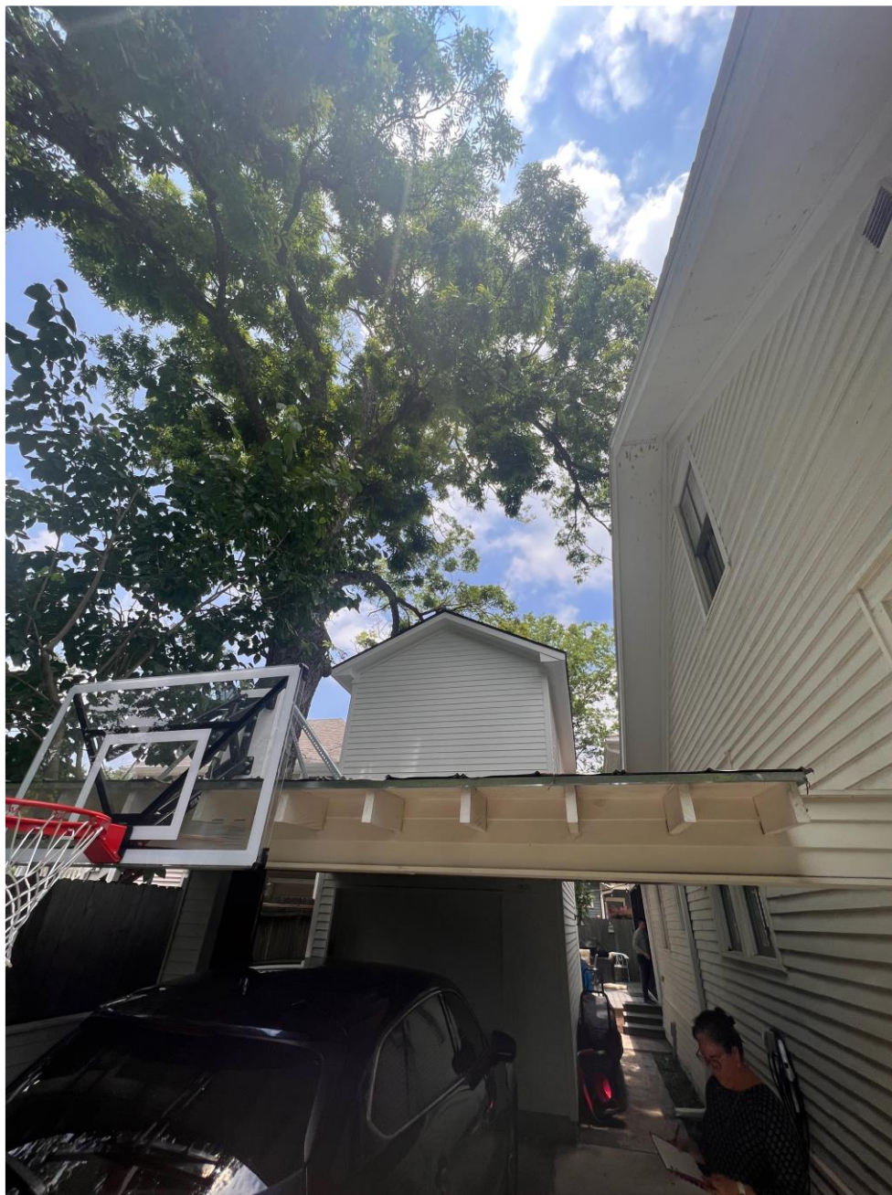
Front of Garage Carport Attached to House
