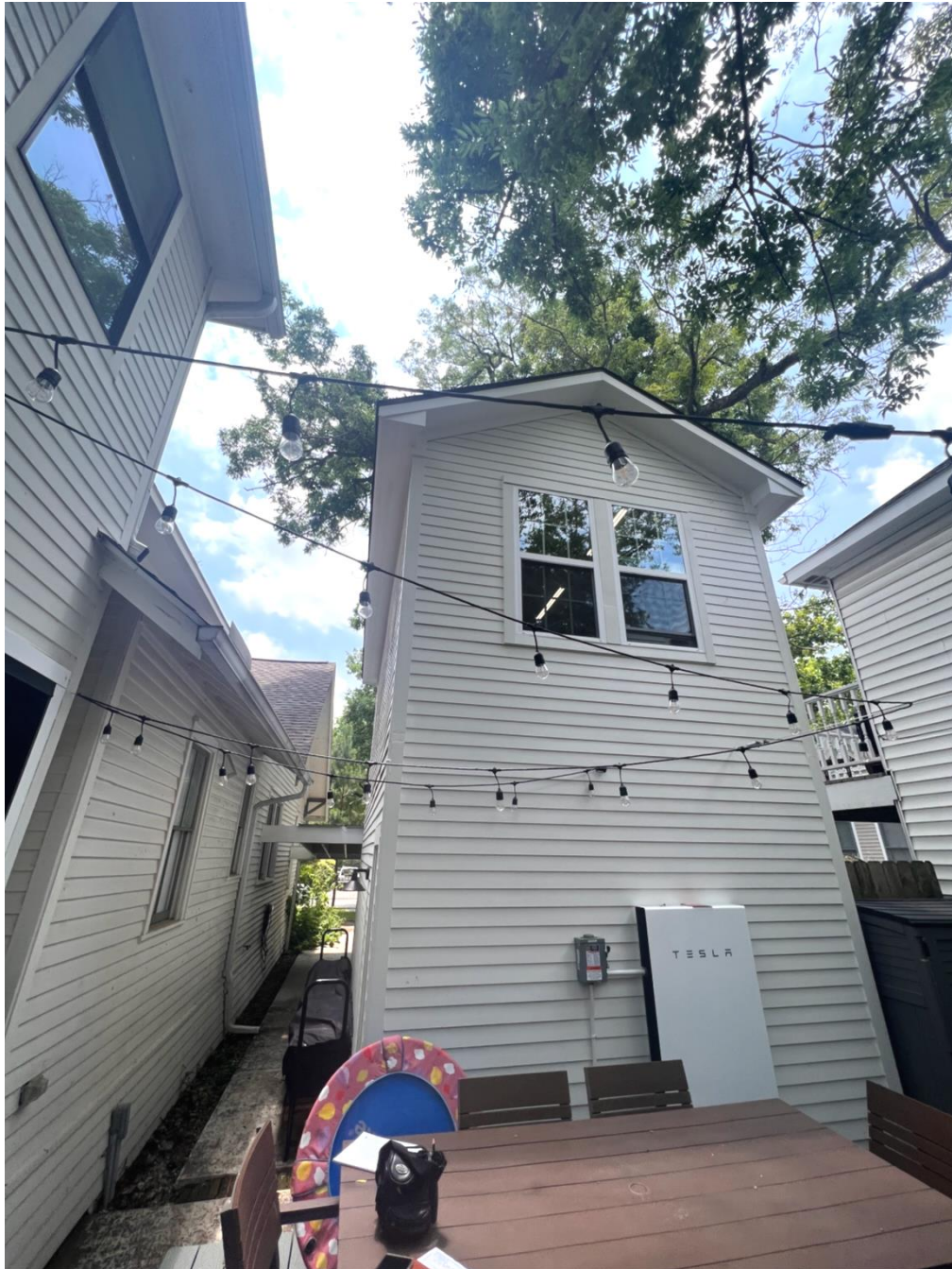
Back of Existing Garage
