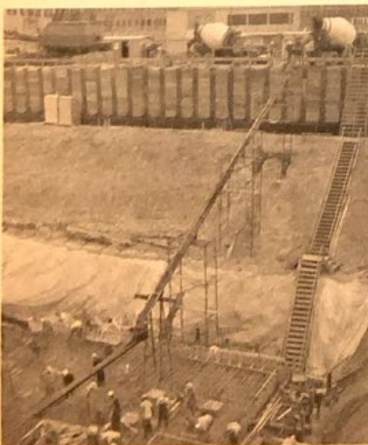
Concrete is being placed here on the foundation mat.
