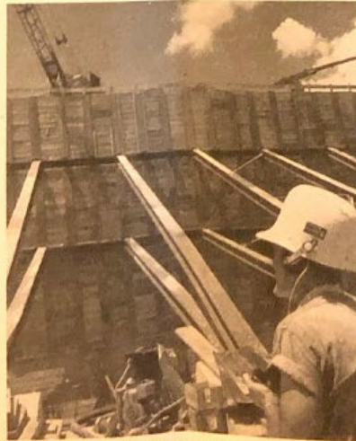
Equipment is lowered by crane into foundation excavation.
