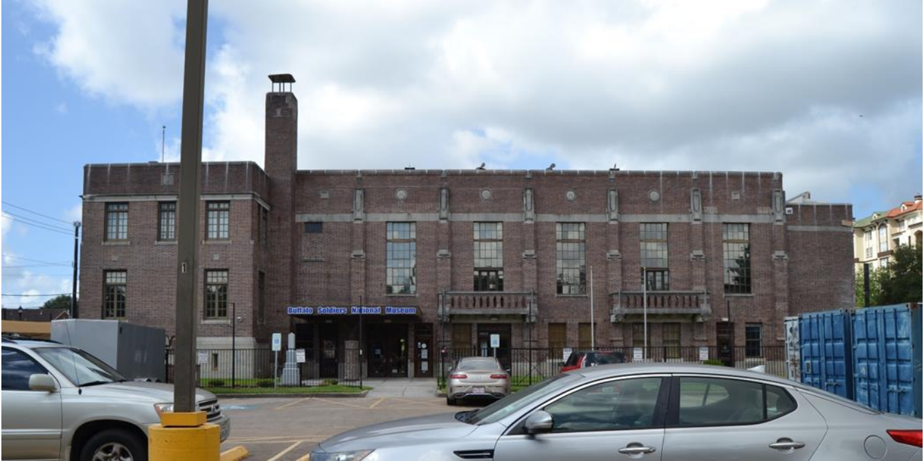
Photo 3. Side northeast façade. Camera facing southwest.
