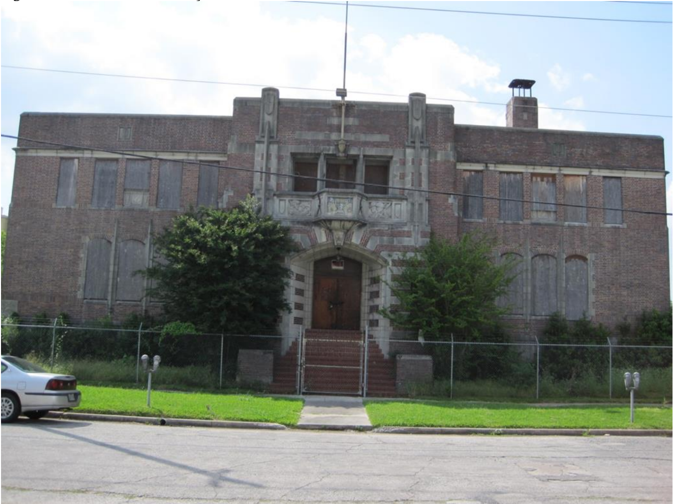
Figure 11. The front southeast façade in 2010. Source: Texas Historical Commission.
