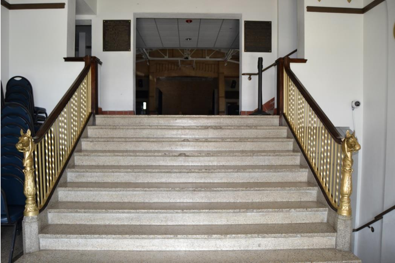
Photo 18. Terrazzo stairs leading from front wing historic-period entrance lobby to the drill hall. Camera facing northwest.
