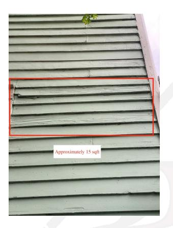
The wood siding in the specified area has been compromised by water damage.
