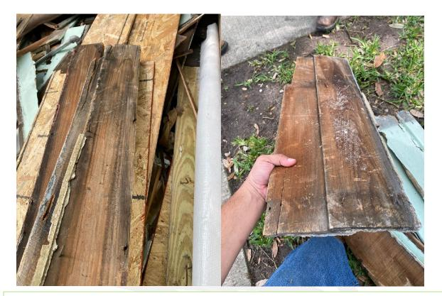
As we attempted to remove the siding, to maintain the integrity of the original wood, the nails were splitting the siding.
