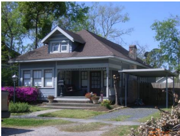
723 Arlington Street – Contributing – 1910 (across street)
