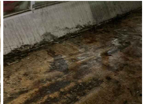
Back porch rear wall and floor
