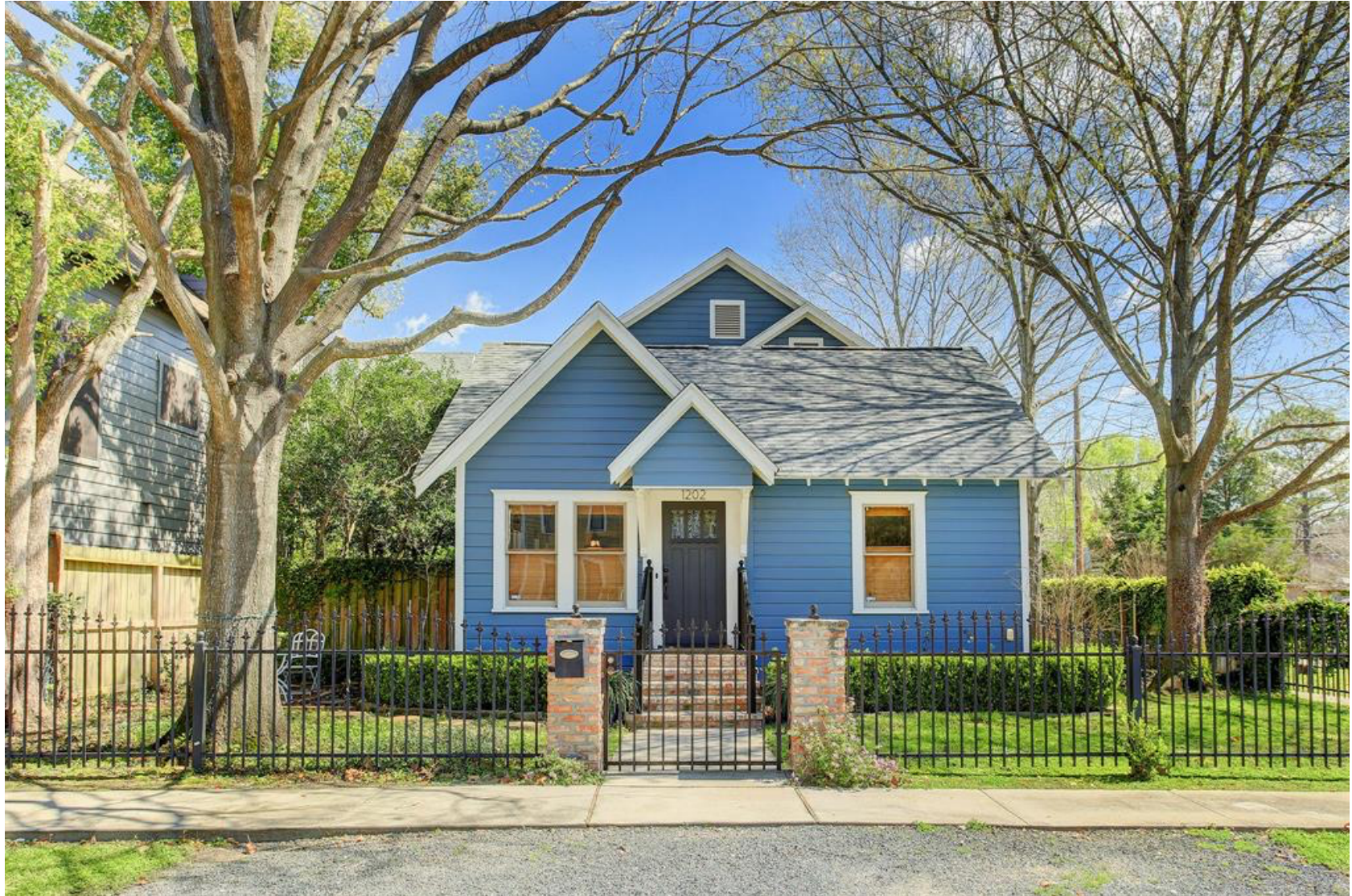
1202 ASHLAND STREET FRONT DOOR FACING WEST
