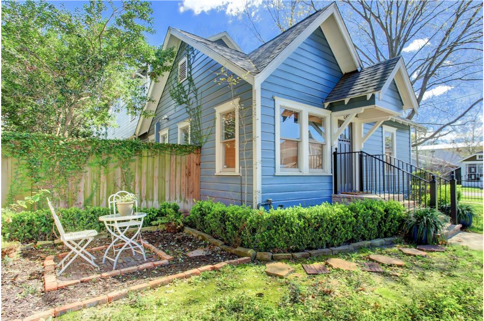
1202 ASHLAND STREET FRONT DOOR FACING WEST
