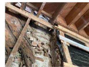
4. Top plate condition at east side of existing fireplace
