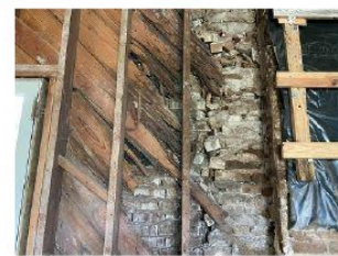
3. Wall condition at east side of existing fireplace
