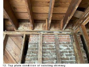
12. Top plate condition of existing chimney
