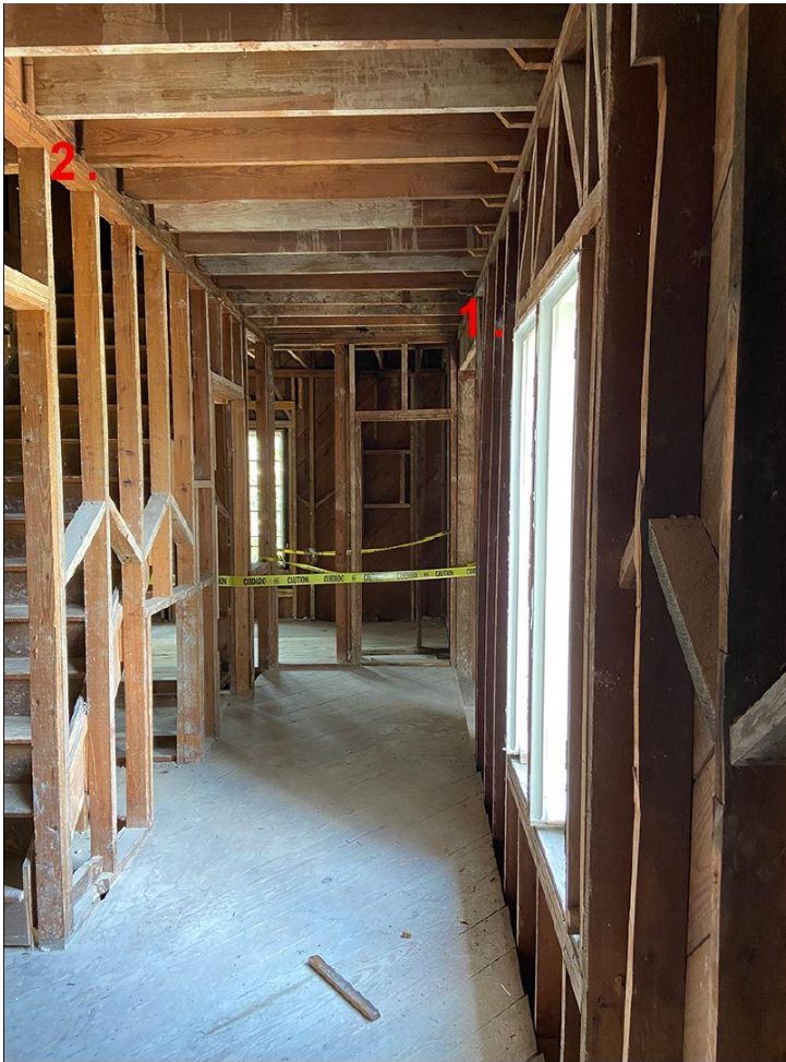
Laser point is aligned with bottom plate below. Top of wall is currently +/-7" out of plumb.
