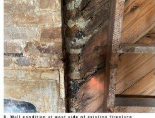
6. Wall condition at west side of existing fireplace
