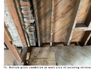
13. Bottom plate condition at west side of existing chimney
