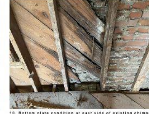
10. Bottom plate condition at east side of existing chimney
