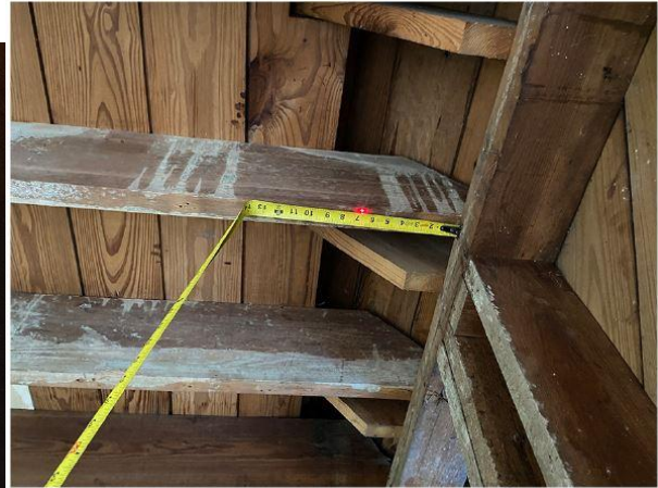
Laser point is aligned with bottom plate below. Top of wall is currently +/-7" out of plumb.
