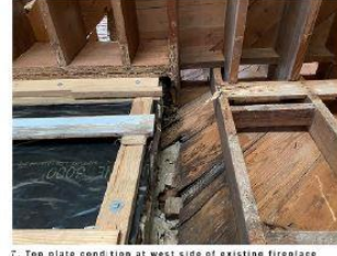
7. Top plate condition at west side of existing fireplace
