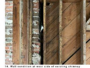
14. Wall condition at west side of existing chimney
