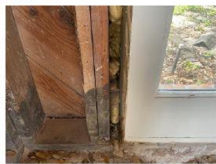
1. Bottom plate condition at east side of existing Sun Room
