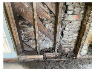
2. Bottom plate condition at east side of existing fireplace
