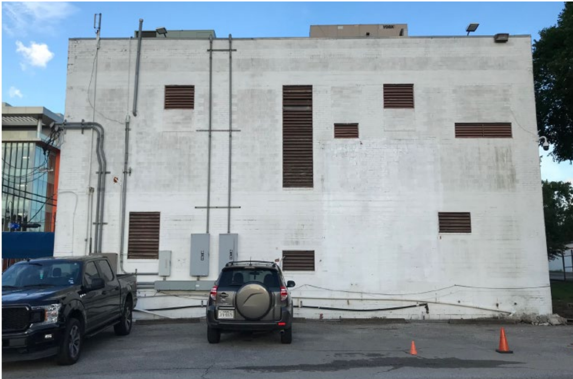
West Elevation, partially infilled historic openings on wood louvered screens
