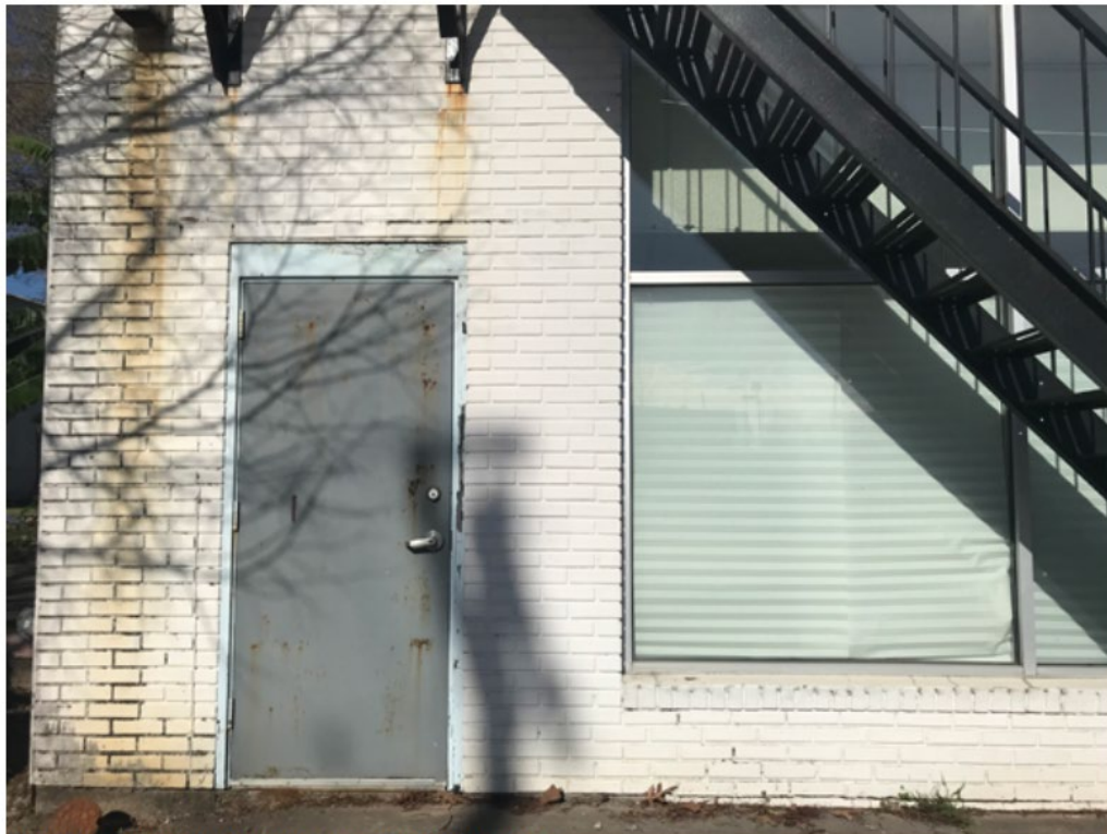
East Elevation Detail, storefront windows from the 2000s and steel door
