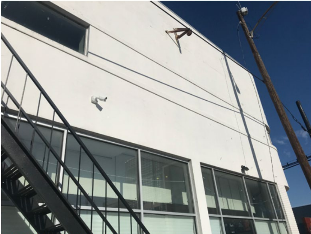
East Elevation Detail, fixed windows at second level
