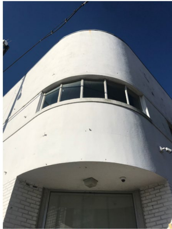
Northeast Corner Detail, fixed windows at second level
