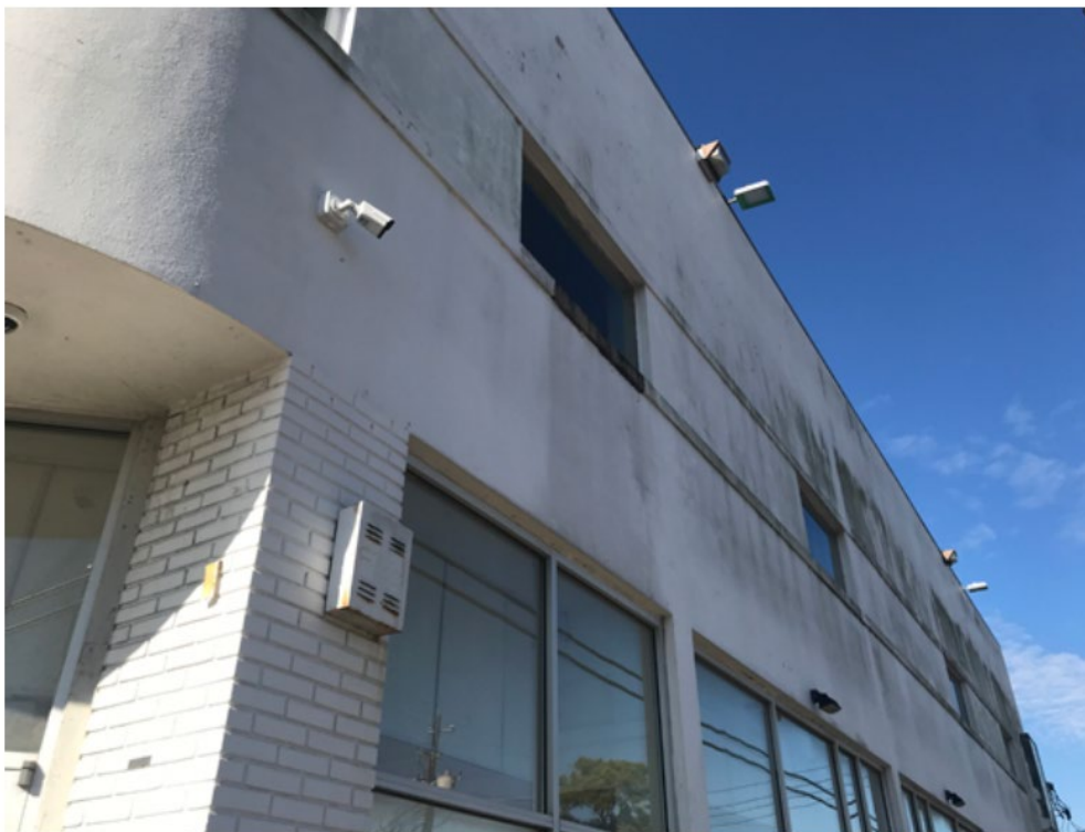
North Elevation Detail, fixed windows at second level
