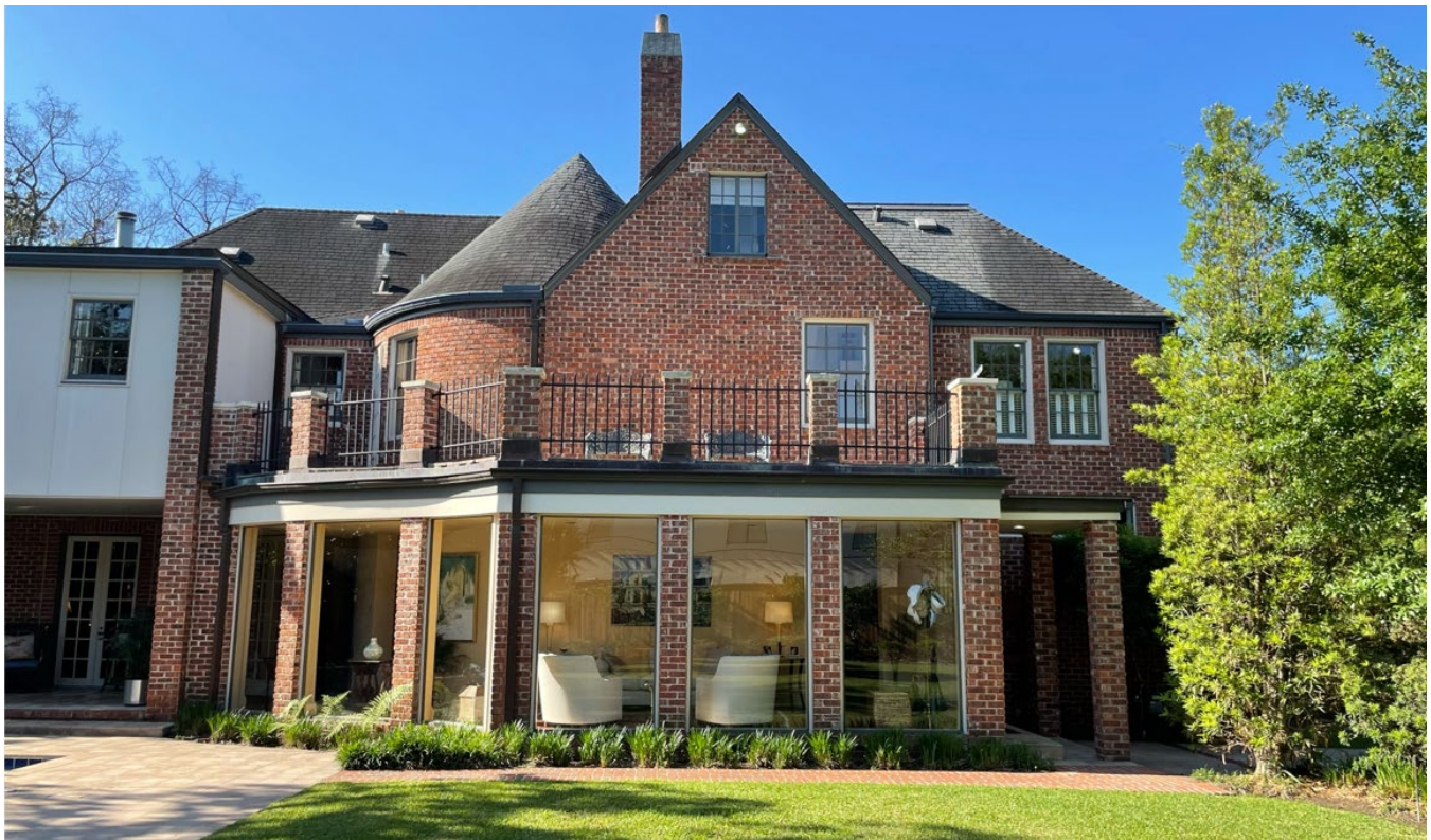
Porch enclosed/alterd after c. 1980
