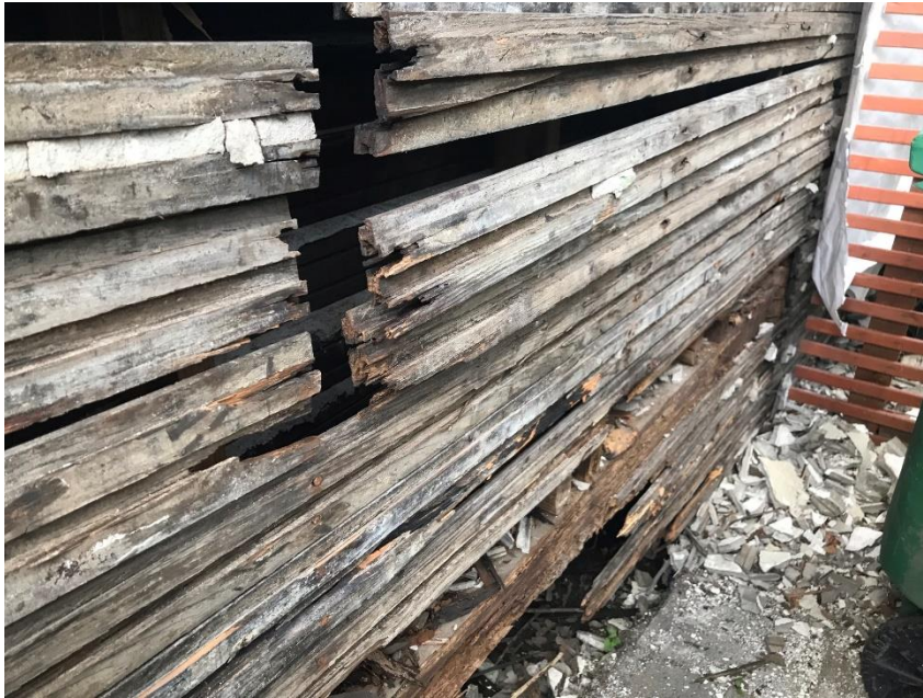
Figure 8- Exposed wood lath from the removal of the original stucco.
