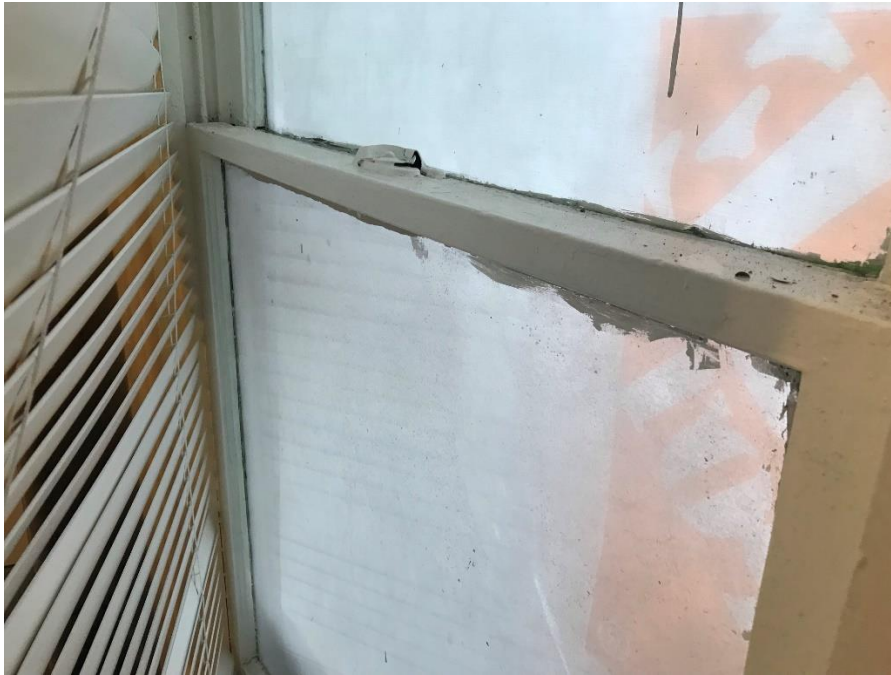
Figure 6 - existing windows appear restorable.
