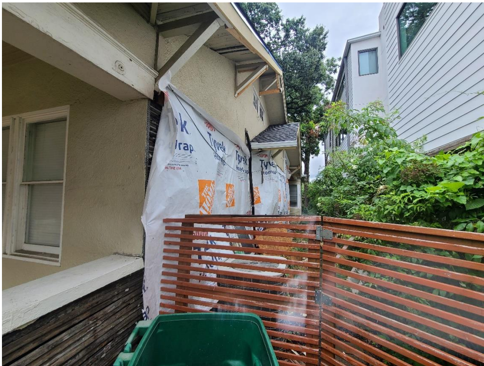
Figure 4 - Staff Photo 2 July 2021-view down East side where work has started
