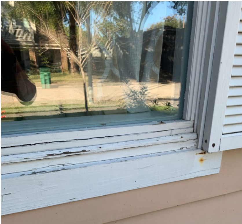
WINDOW B (FRONT ELEVATION) – TO REMAIN, GLASS REPLACED, REPAIR
