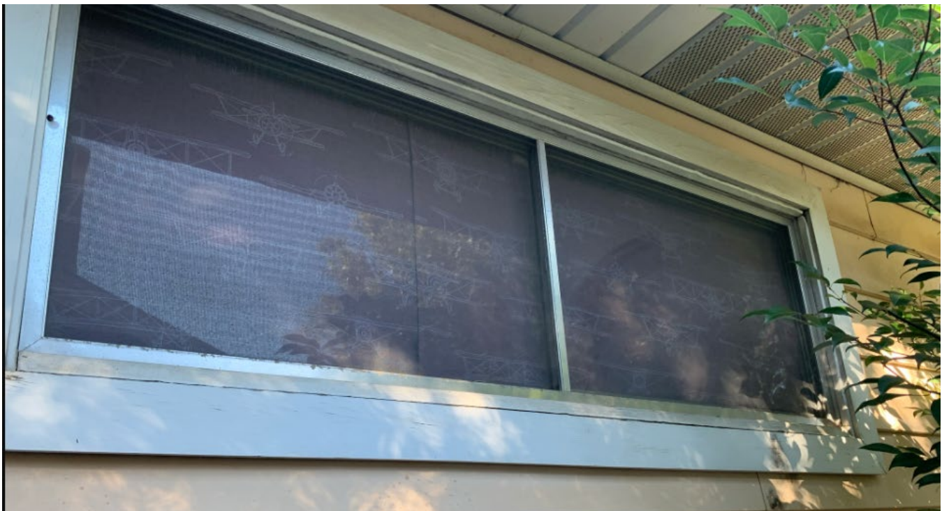
WINDOW J (FRONT LEFT ELEVATION/SIDE) REPLACEMENT ALUMINUM – KEEP OPENING, REPLACE WITH WOOD WINDOW
