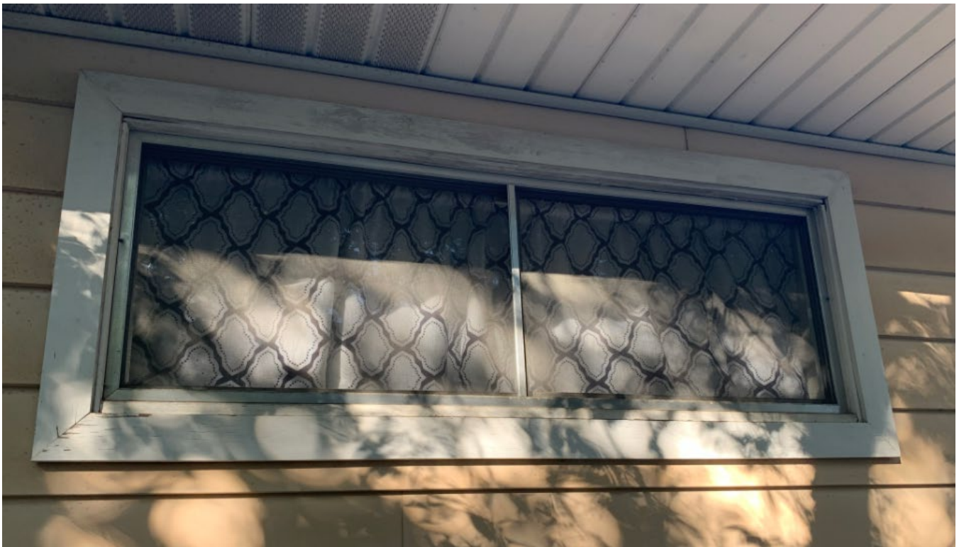
WINDOW H (LEFT ELEVATION REAR, REPLACEMENT ALUMINUM) PROPOSED REPLACEMENT WITH DOUBLE HUNG, PAIRED WOOD WINDOW, NEW OPENING
