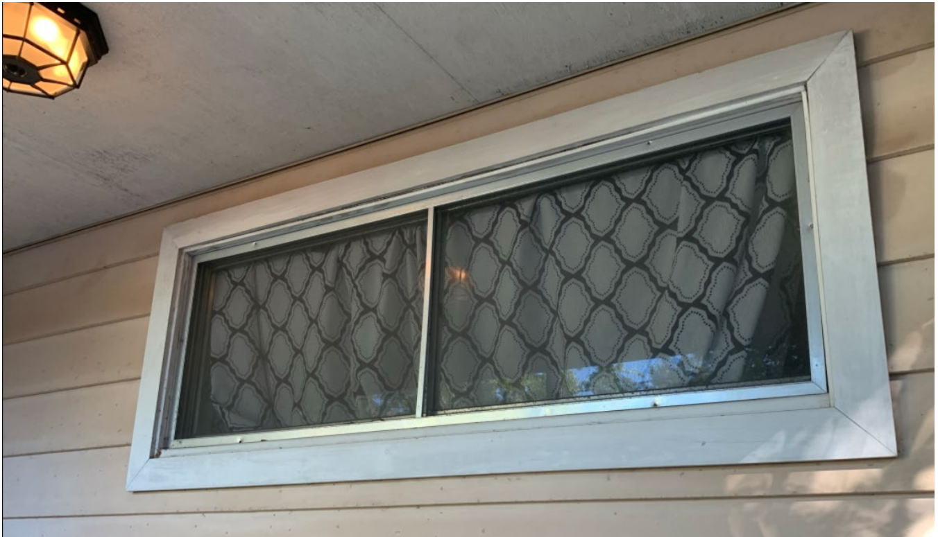
WINDOW H (LEFT ELEVATION REAR, REPLACEMENT ALUMINUM) PROPOSED REPLACEMENT WITH DOUBLE HUNG, PAIRED WOOD WINDOW, NEW OPENING
