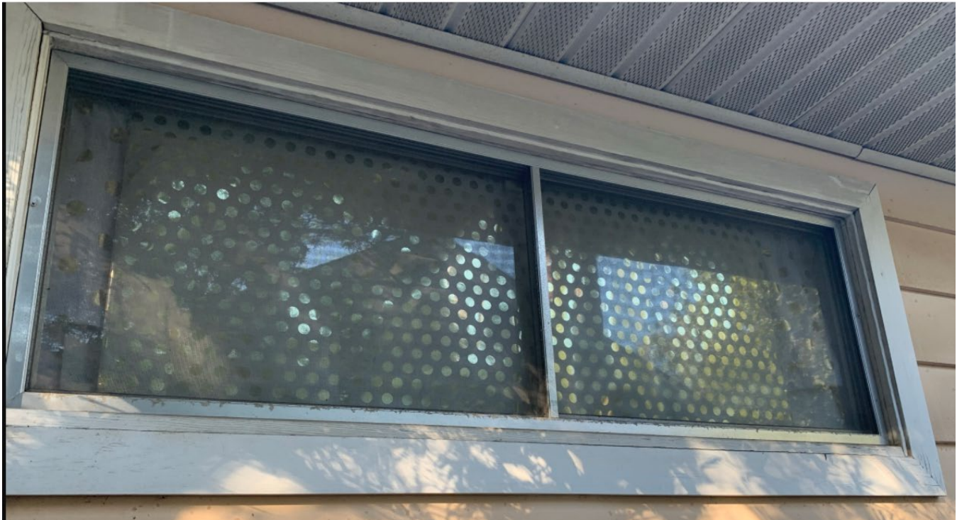
WINDOW J (FRONT LEFT ELEVATION/SIDE) REPLACEMENT ALUMINUM – KEEP OPENING, REPLACE WITH WOOD WINDOW
